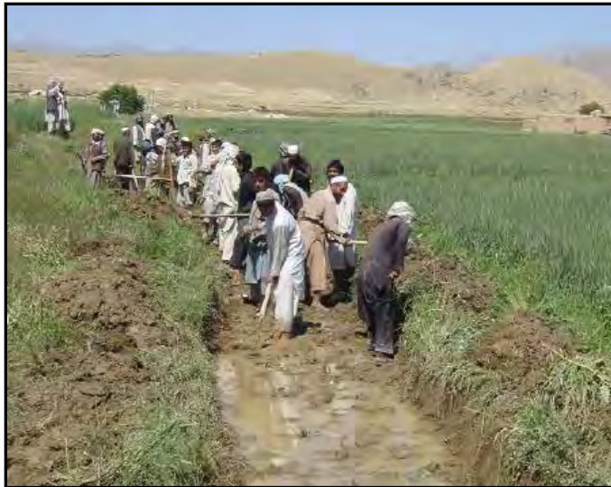
Photo 1: Canal Cleaning in Mibarchakot District, Kabul
