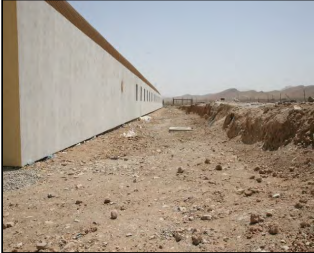
Photo 9: Problematic Grading next to K-Span 3
