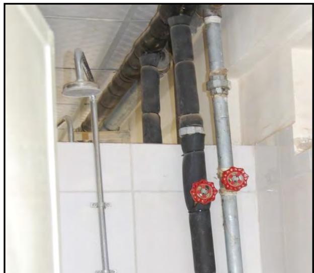
Photo 7: Insubstantial Shower Heads at Mazar-e-Sharif
