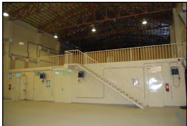
Photo 4: Vehicle Maintenance Building at Mazar-e-Sharif
