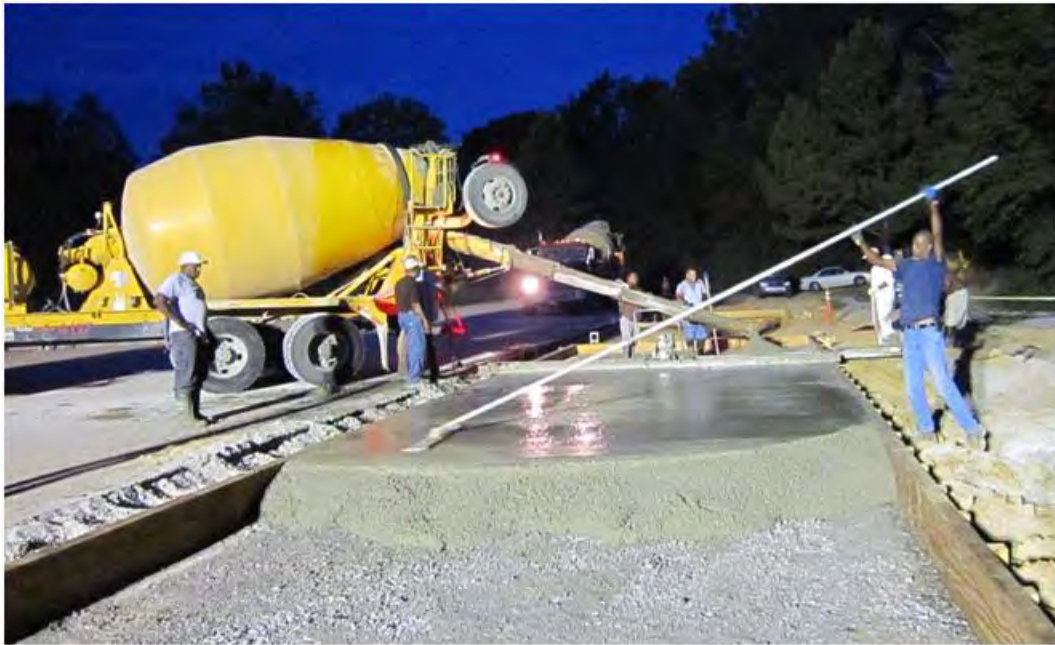
Figure 12. PCC placement.
