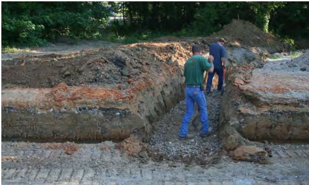
Figure 7. Drainage construction.
