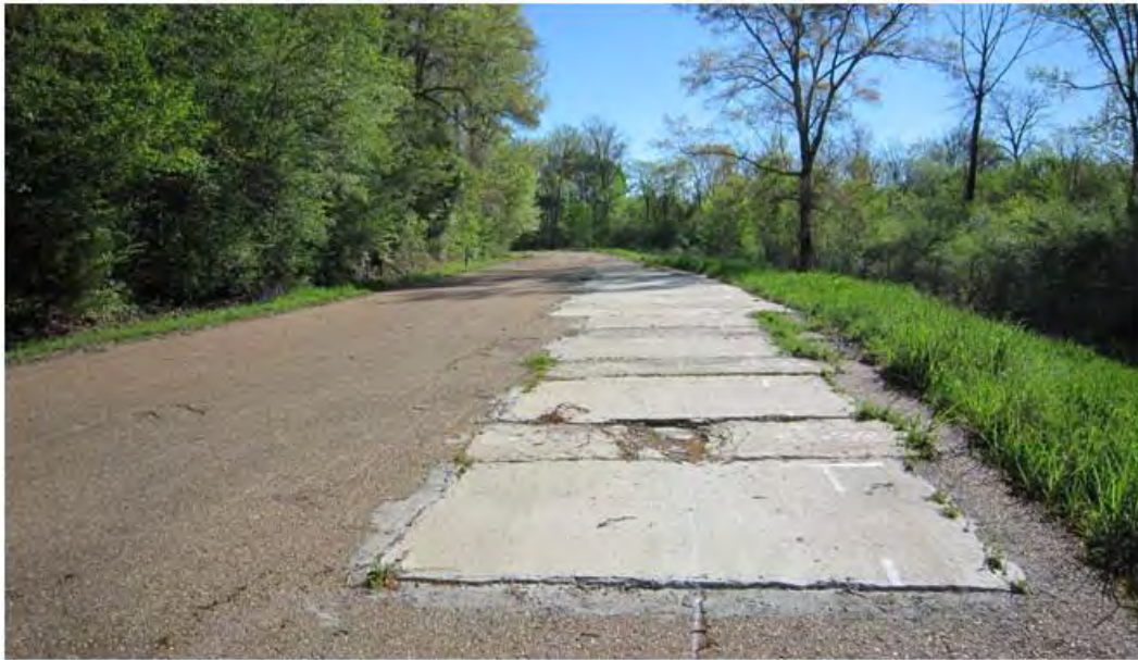
Figure 15. The flowable fill section is shown here on the right and was located within the Forest Service Road.
