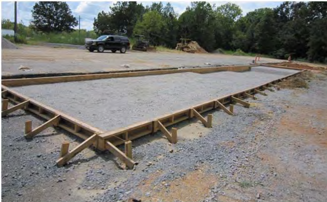
Figure 11. Forms for the PCC placement.
