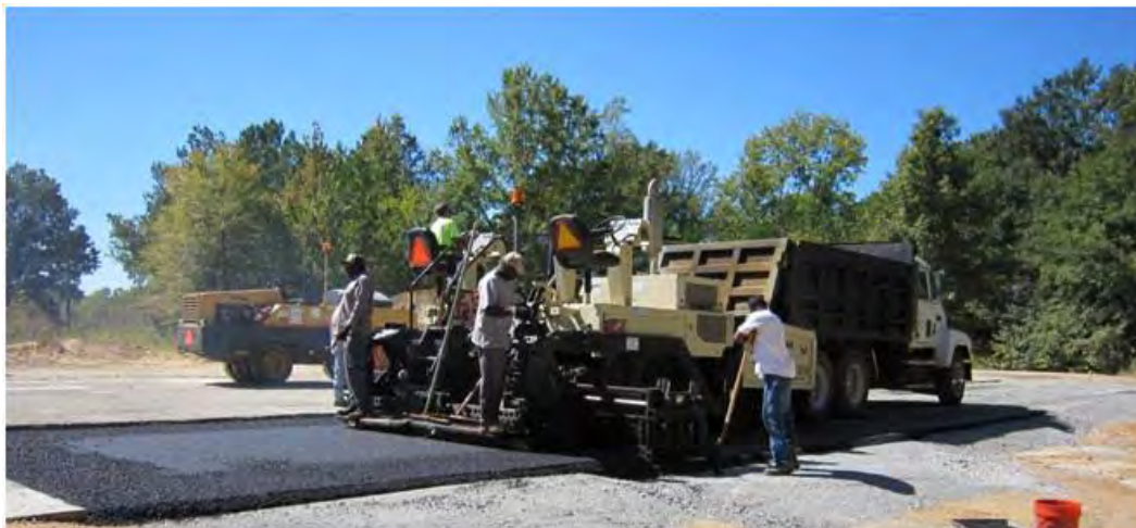
Figure 8. Asphalt placement.
