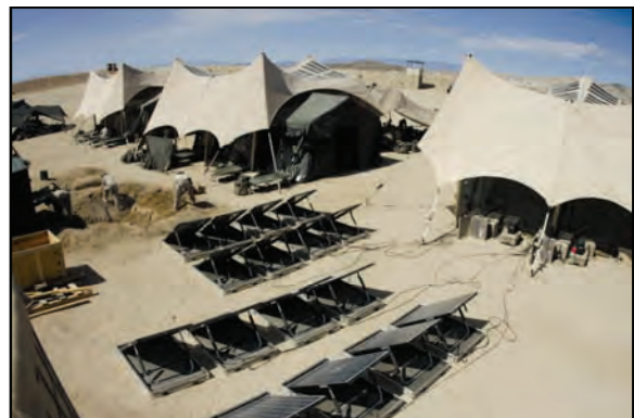
Solar array at a forward-operating base
