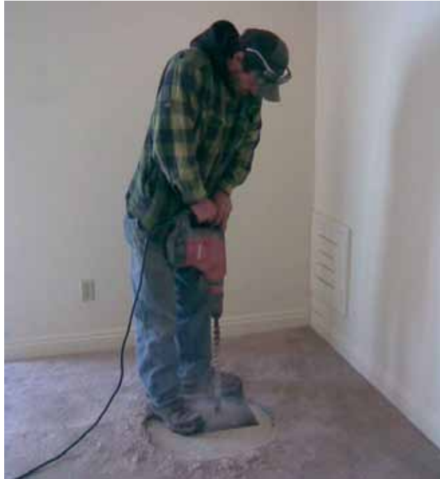
Figure 18. Drilling 1-in. holes.
