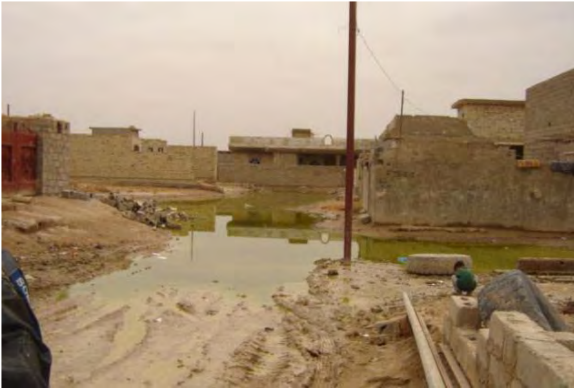
Figure 1—Raw Sewage in Falluja Streets
