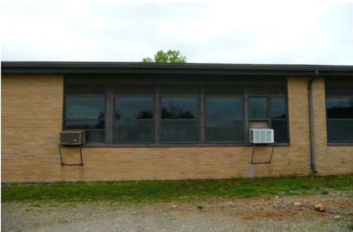
Photo 18. Typical replacement one-over-one double-hung windows on the addition portion of the cafeteria.
