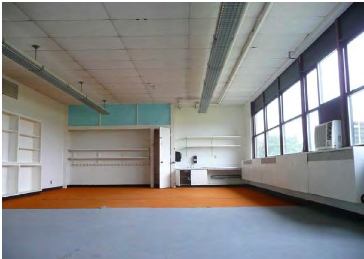
Photo 94. Interior of Classroom No. 16.
