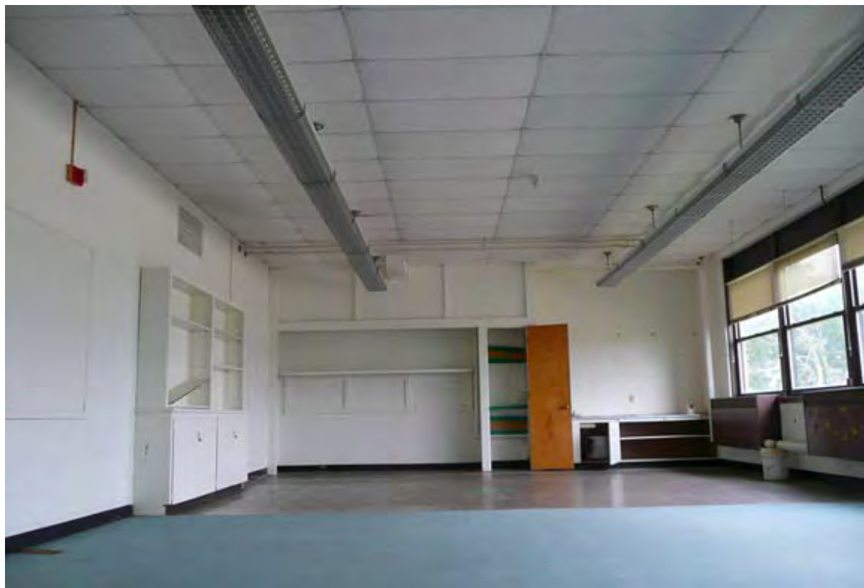
Photo 82. Interior Classroom No. 13.
