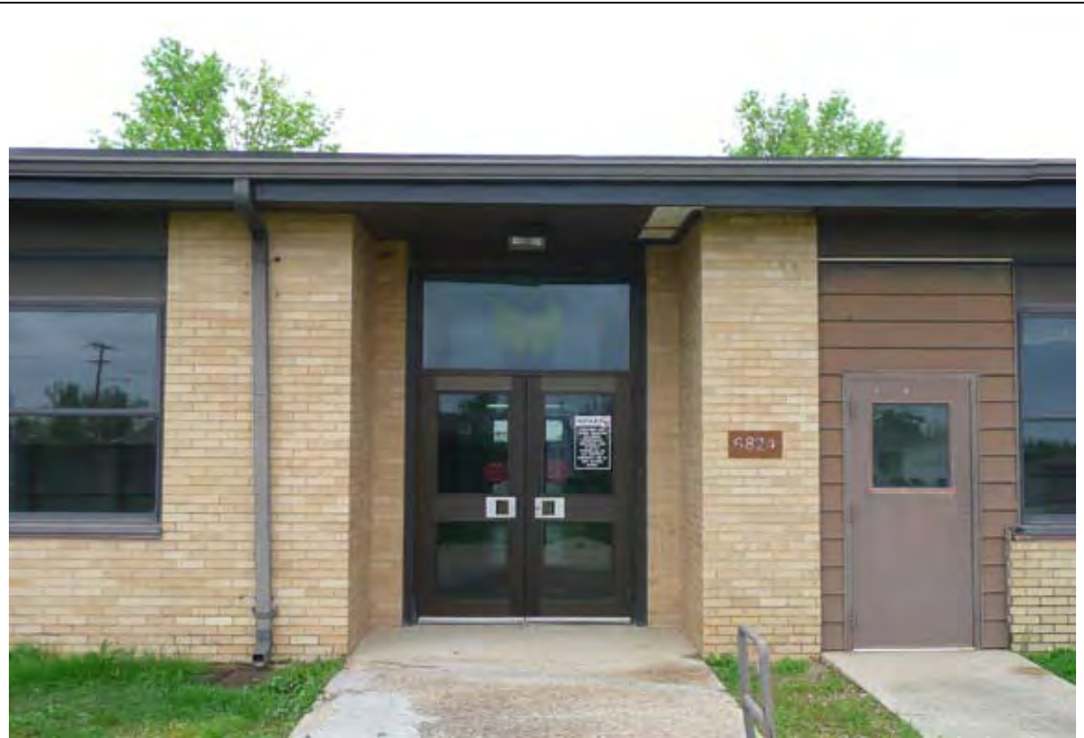
Photo 25. Main entry on the south elevation.
