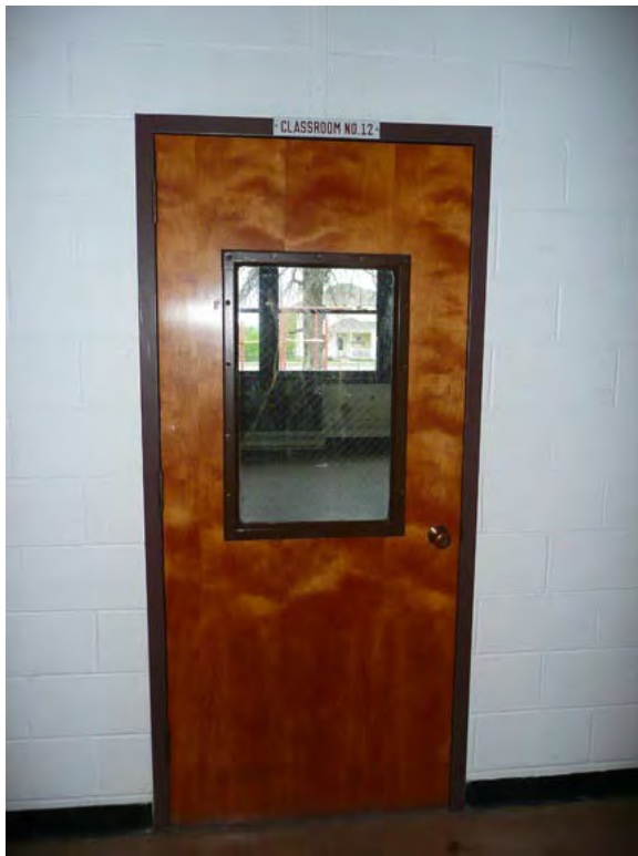
Photo 75. Classroom No. 12 replacement door.
