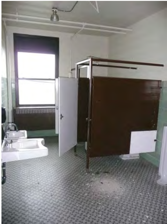
Photo 130. Original mosaic tile floor and glazed tile walls in Boys' Toilet No. 24.
