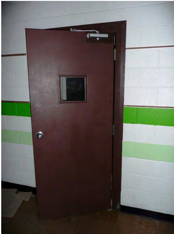
Photo 103. Newer metal door leading into the kitchen.
