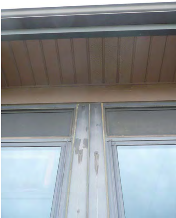
Photo 20. Replacement aluminum soffit and gutters.
