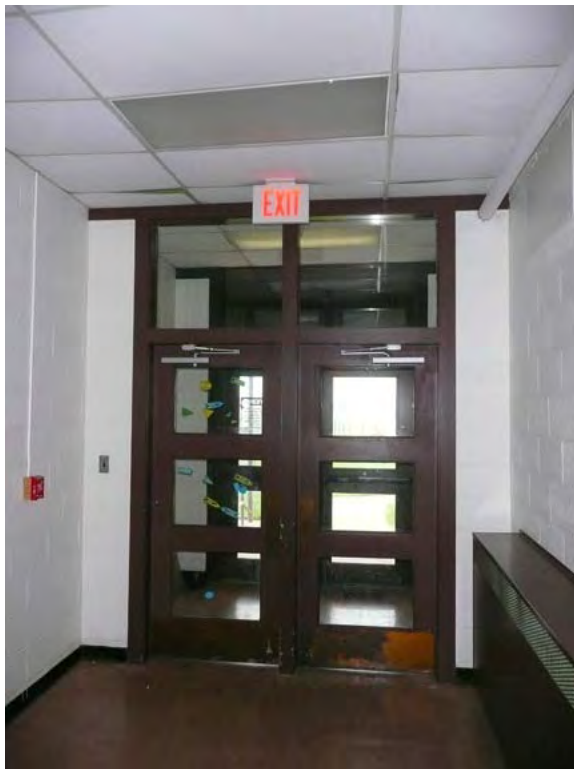
Photo 78. Original metal vestibule doors and transom located at the east end of the corridor.
