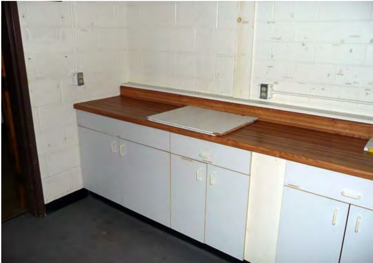
Photo 59. Replacement cabinets in Health Room No. 5.
