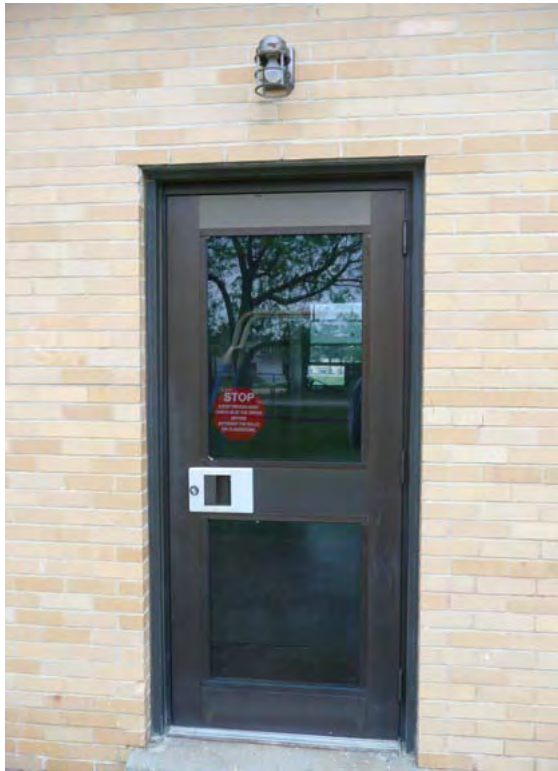
Photo 17. Typical replacement entry door.
