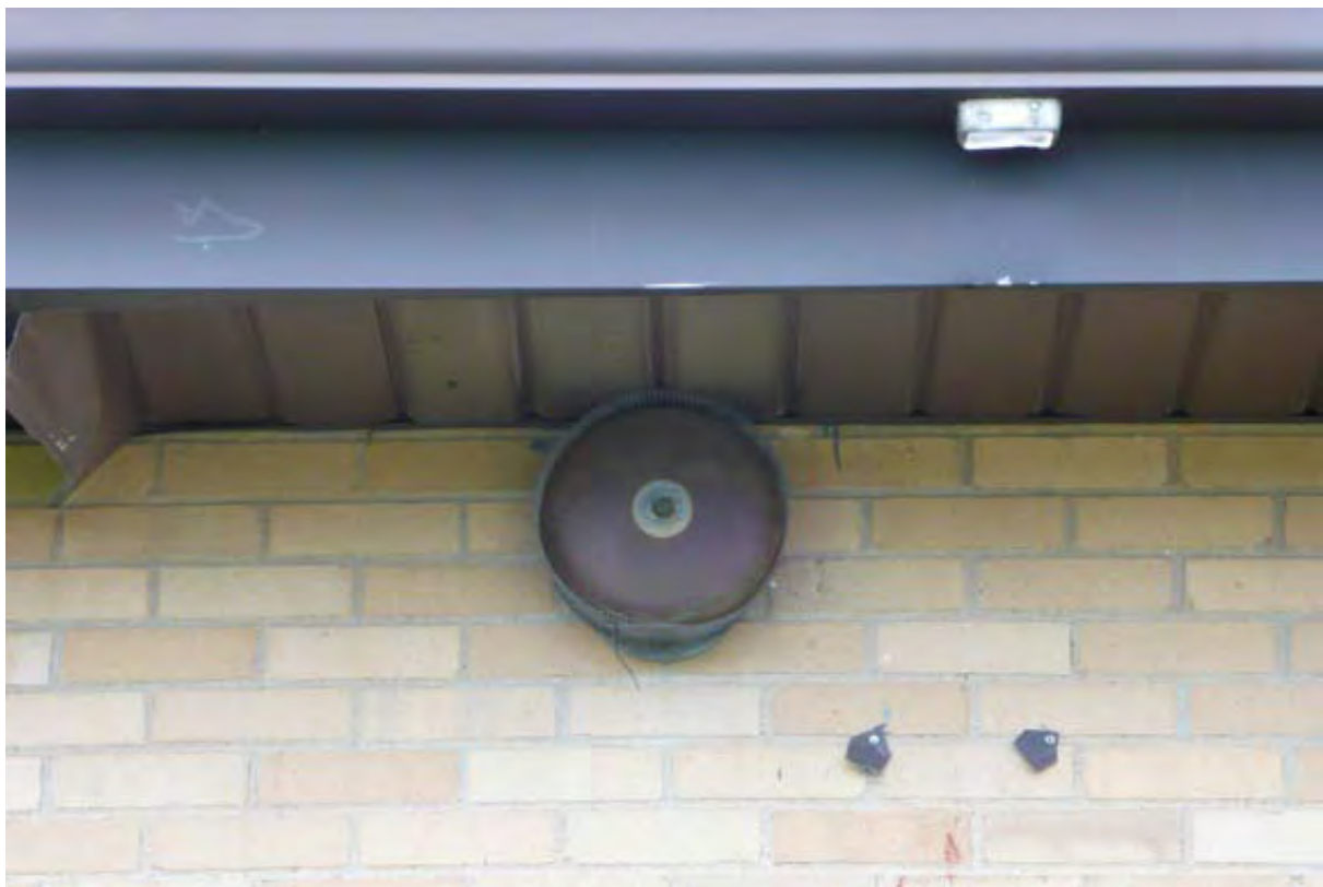
Photo 26. Bell and replacement metal soffit and fascia.
