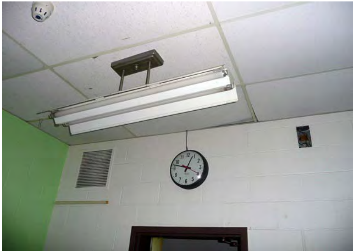
Photo 61. Replacement light fixture in Office No. 6.
