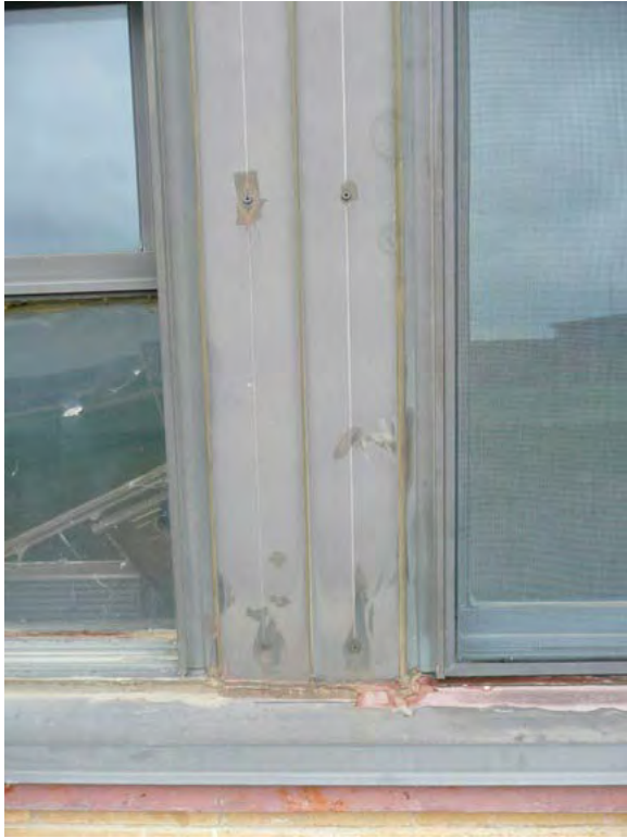
Photo 19. Close-up of replacement window and windowsill.
