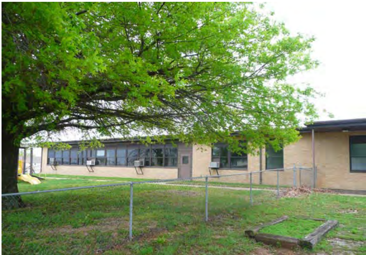
Photo 2. Left side of the north elevation.
