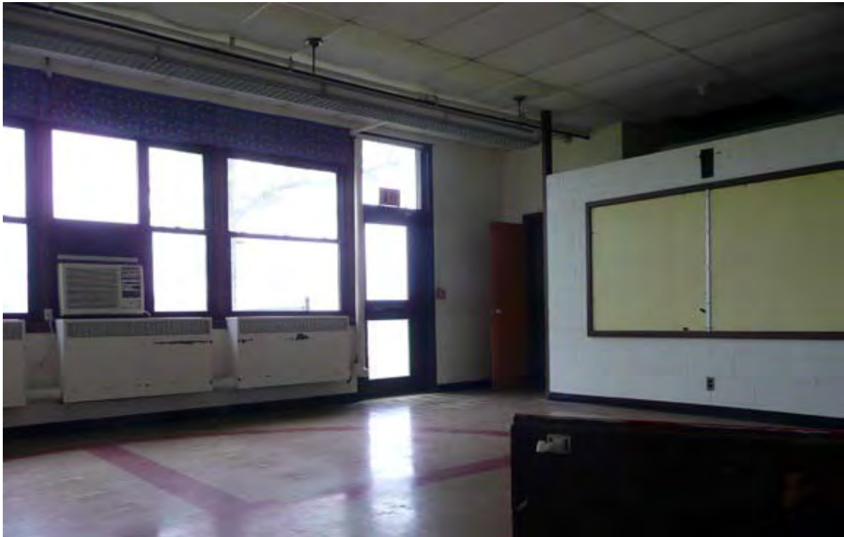
Photo 122. Interior of Primary Room No. 23.
