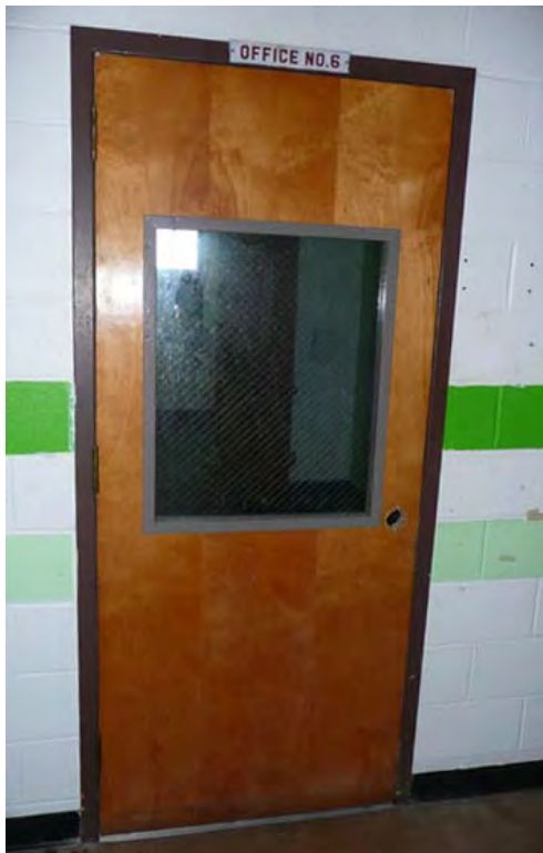
Photo 60. Office No. 6 replacement door.
