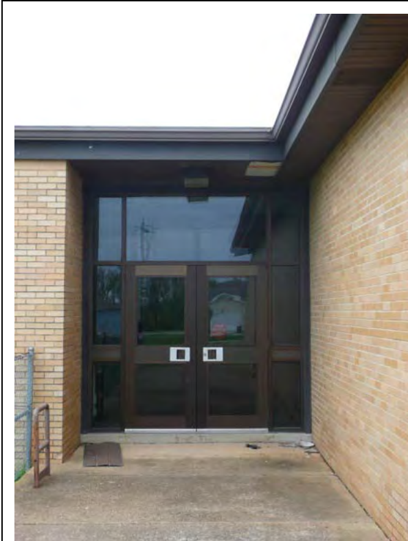
Photo 15. Close-up of replacement doors, transom, and sidelights on the left side of the south elevation.
