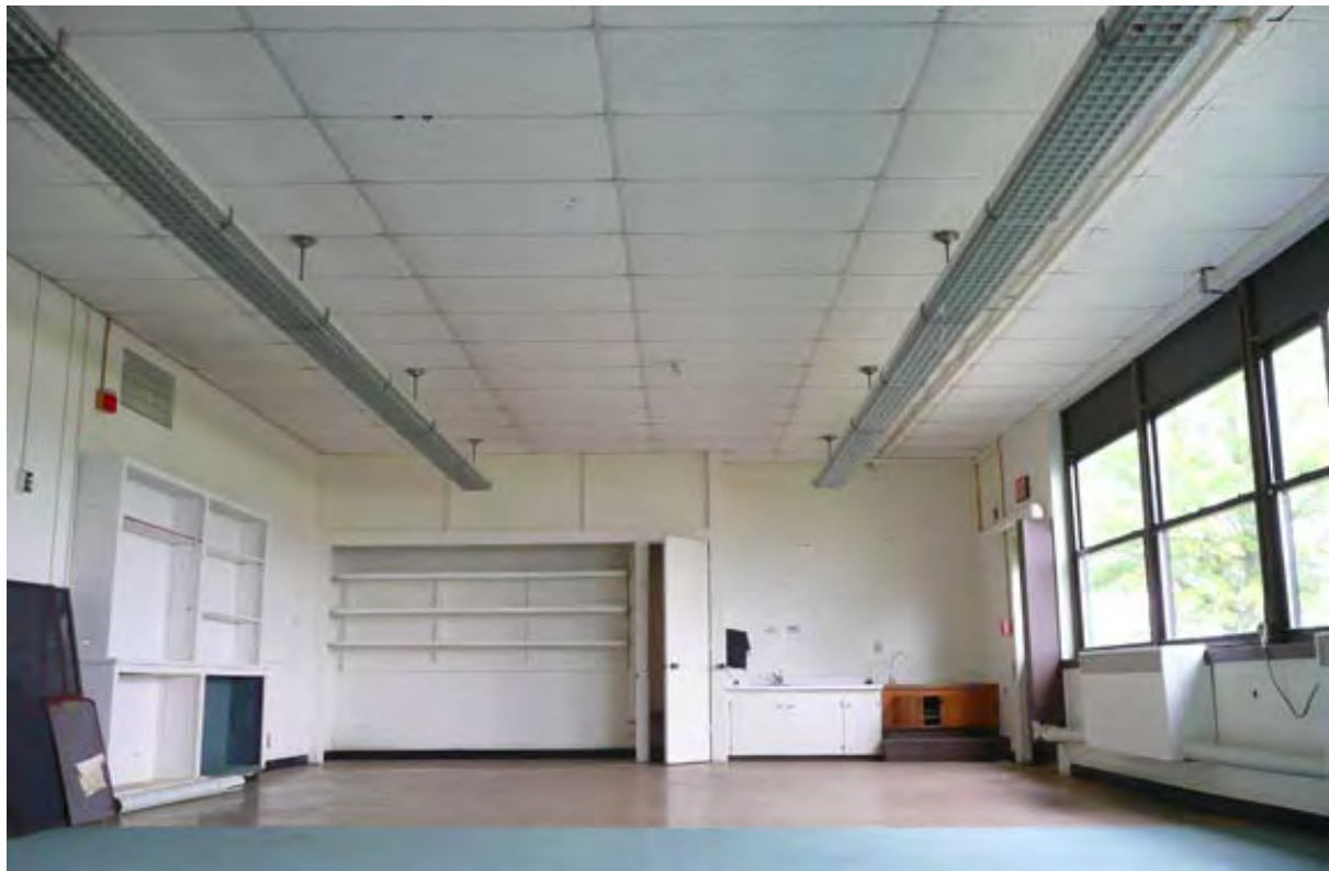
Photo 71. Interior of Classroom No. 11.
