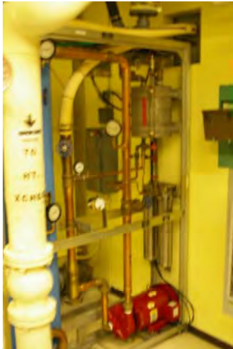
Fig. 11: Vacuum switches at LORSTA Tok Antenna Coupler Room
