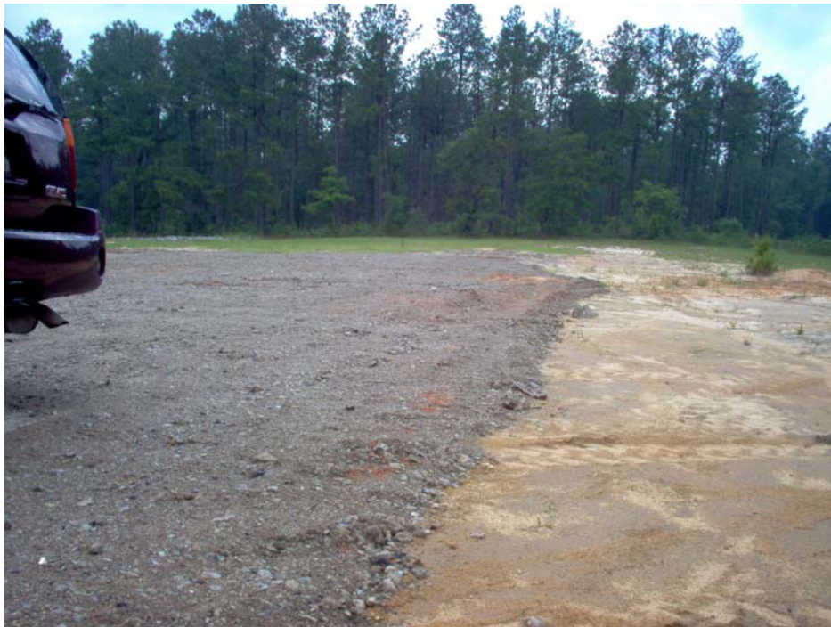
Figure 9. Crushed concrete as paving material at Fort Jackson.
