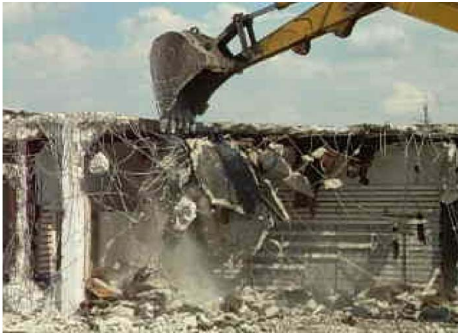
Figure 4. Mechanical demolition of the Fort Jackson CSB.
