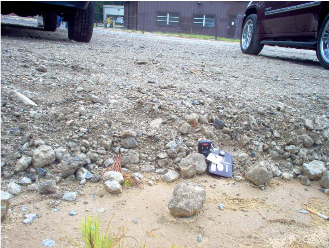
Figure 10. Closeup of paving material.
