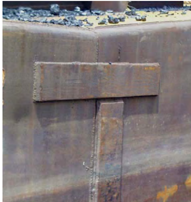
Figure 11. Example of barge protrusions.
