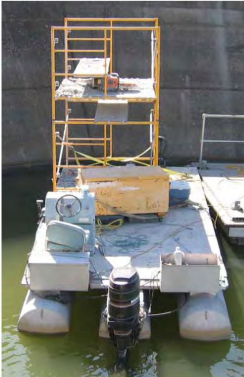
Figure 68. Floating platform for access to repair area.
