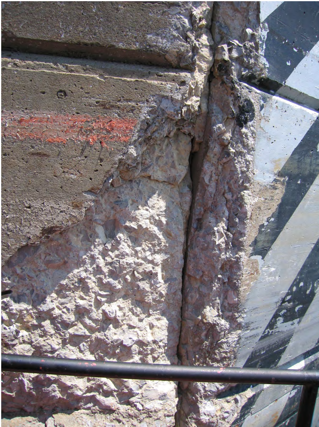
Figure 39. Closeup photo of major concrete damage at the vertical joint to be repaired.
