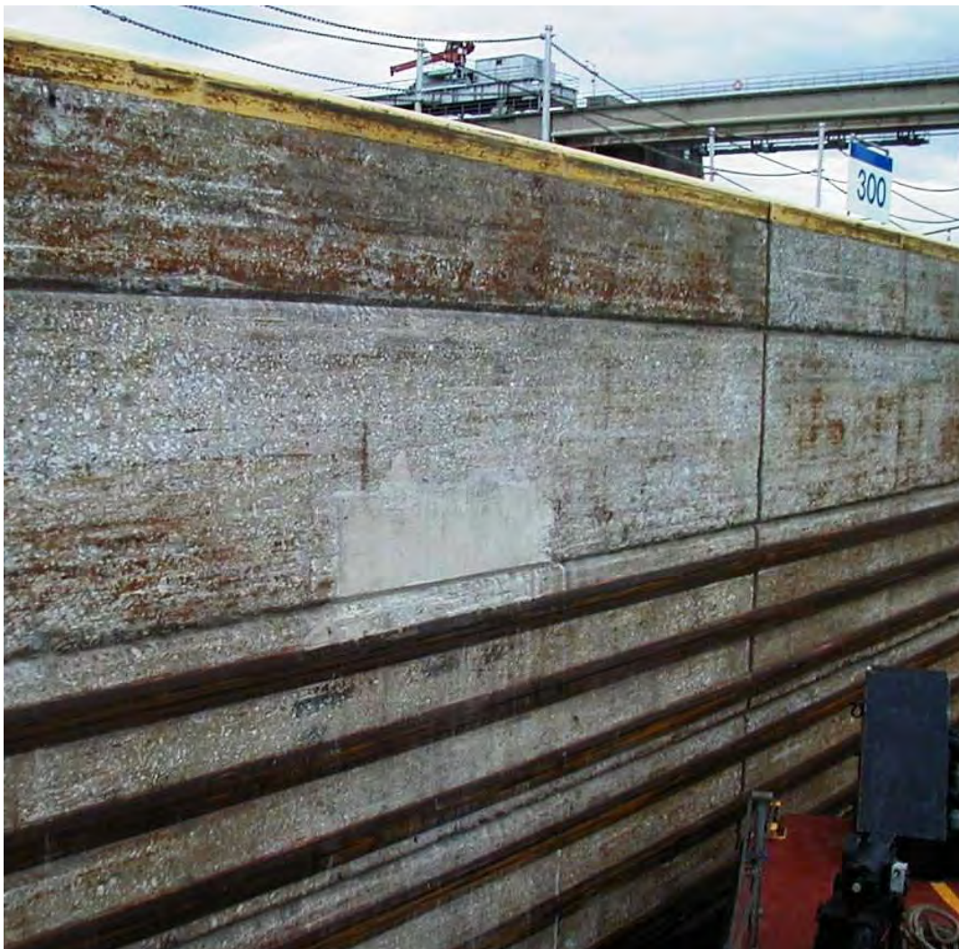
Figure 75. Completed repair of lock approach wall 5 days after placement.
