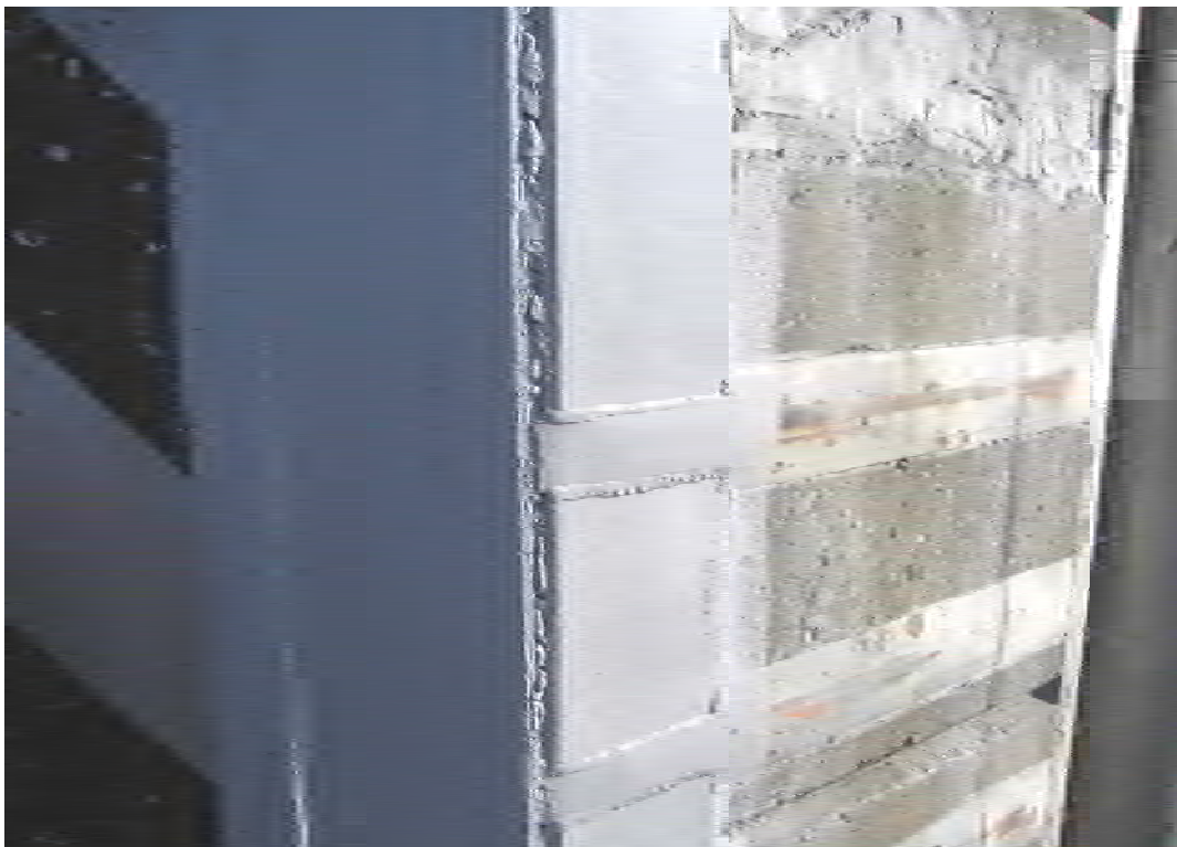
Figure 56. Closeup photo of the 13.5-ft-high by 12-in.-wide top repair steel plate of monolith L-1 on the downstream side of the joint and the 28-in.-high by 12-in.-wide top plate of monolith L-2 on the upstream side of this joint.
