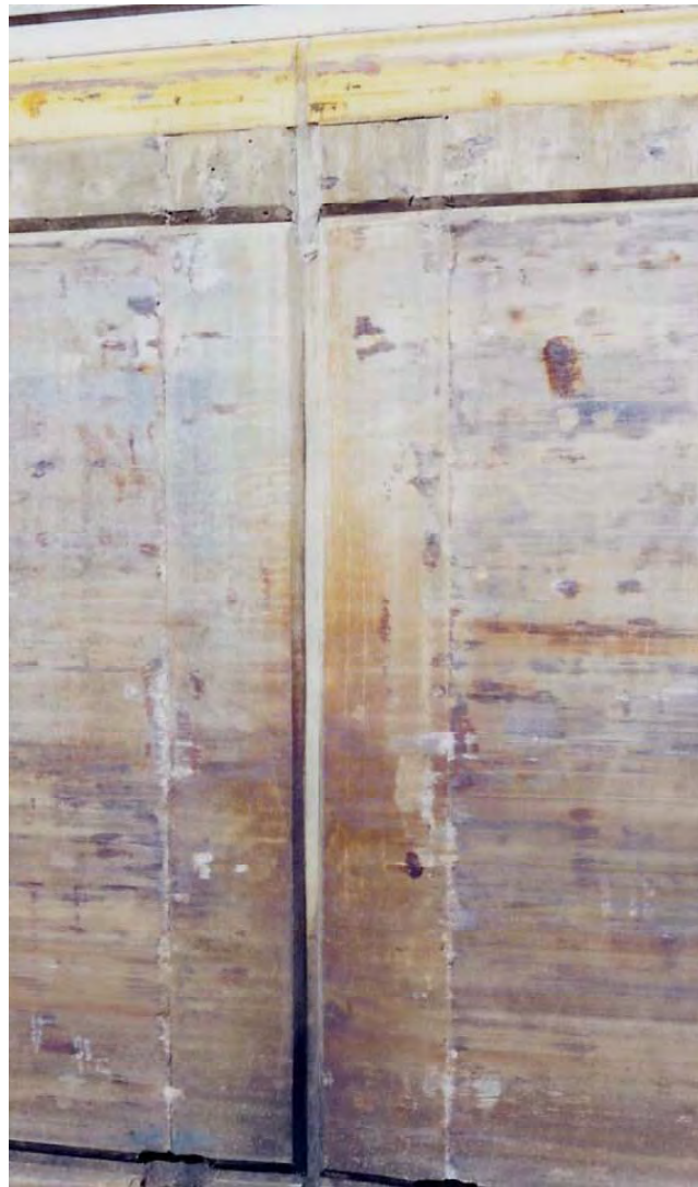
Figure 13. Precast panel joint at Allegheny Lock after four years of service.
