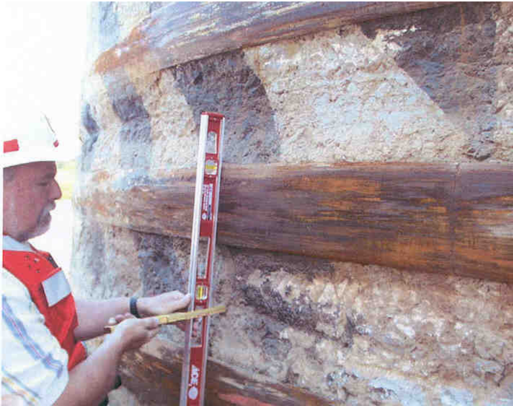
Figure 32. Typical Type V damage, John T. Myers, bullnose.
