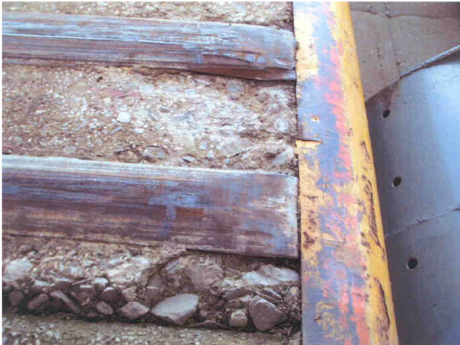
Figure 23. Typical Type II damage, John T. Myers, localized crushing of concrete.
