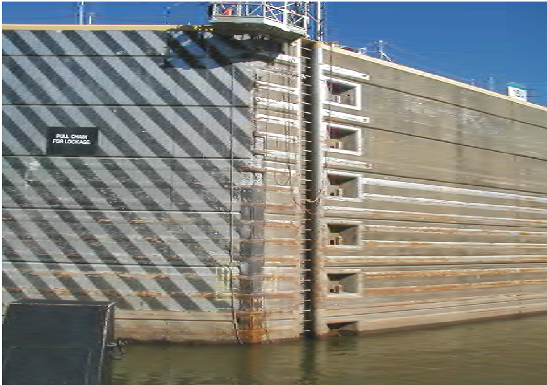
Figure 55. 600-ft chamber lower land-wall approach vertical joint during repair activities.
