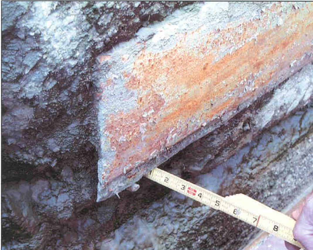
Figure 10. Type I loss of concrete section, John T. Myers.
