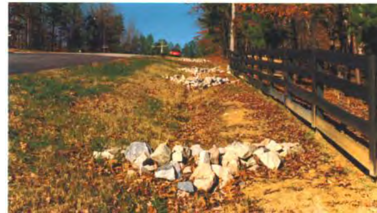
Rip rap check dams along road
