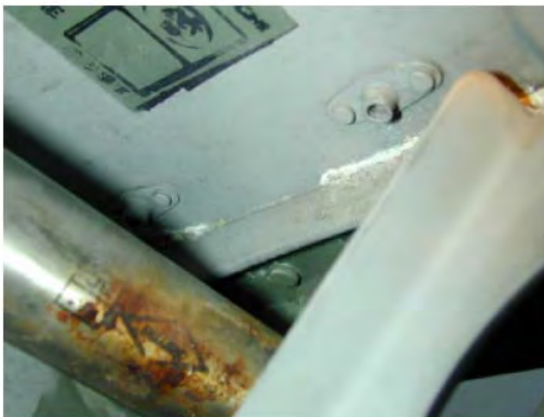
Figure 4-11: Galvanic Corrosion on the MB-339 Attach Fitting.
