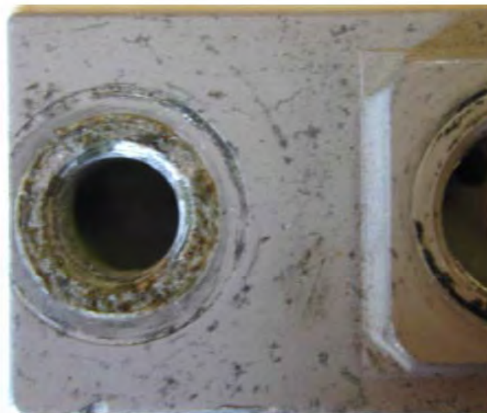
Figure 4-8: Crevice Corrosion on a Tornado.
