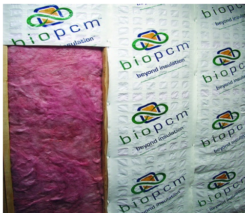
Figure 1. PCM Mats Installed in a Typical Wall
