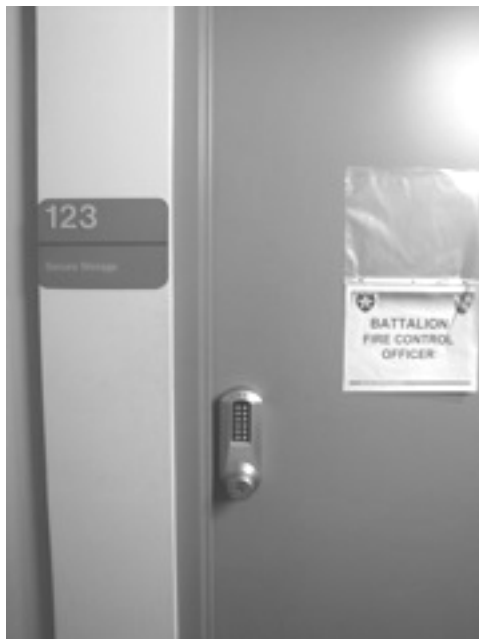
Figure 5: Cipher-locks restrict access to most non-public spaces within newer facilities, including offices, storage areas, secure storage vaults, and SIPR Net rooms. Typically, only the commanding officer of the battalion will have the pass-code for all locked spaces, therefore close contact with the CO in charge of facilities to be surveyed is crucial to reducing logistics time.
