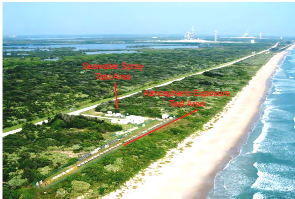
Figure 5-78 NASA Beach Corrosion Test Site
