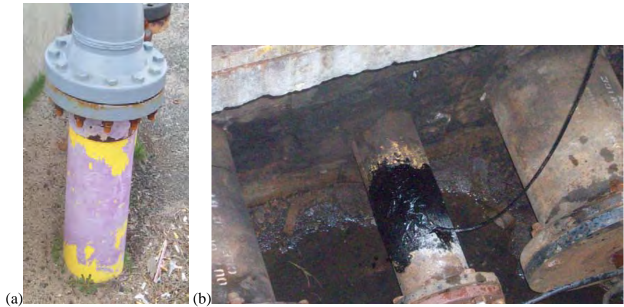
Figure 6. Surface conditions of tested pipe.
