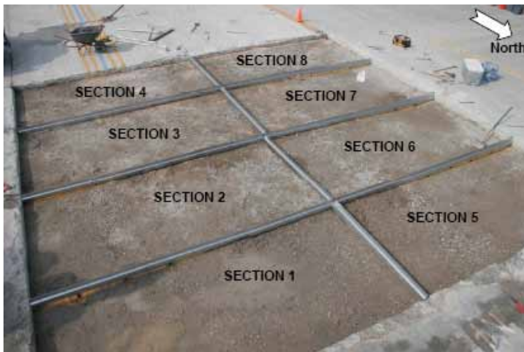
Figure 81. Completion of Crater 4 preparation.
