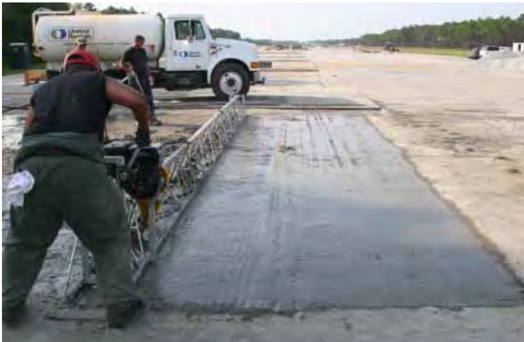
Figure 35. Crater 1, screeding the repair.
