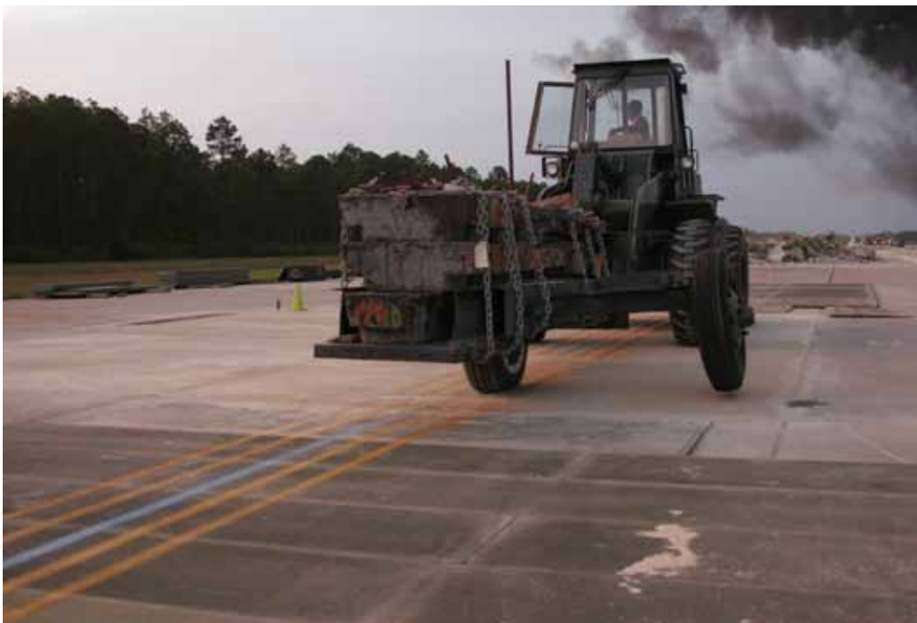
Figure 49. Crater 6, completed repair surface during trafficking.
