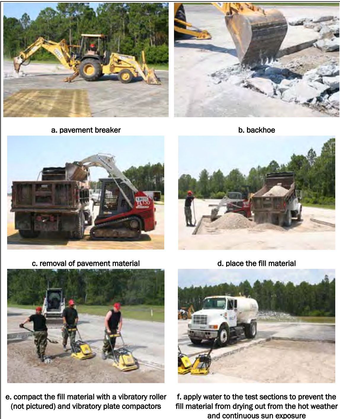
Figure 9. Preparation of the test craters showing the techniques and equipment used to break out and remove existing pavement.
