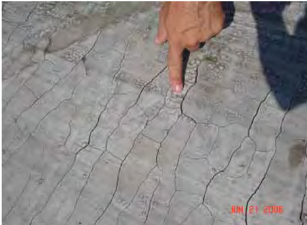
Figure 36. Shrinkage cracks in the surface of the stone and grout repair, Crater 1.
