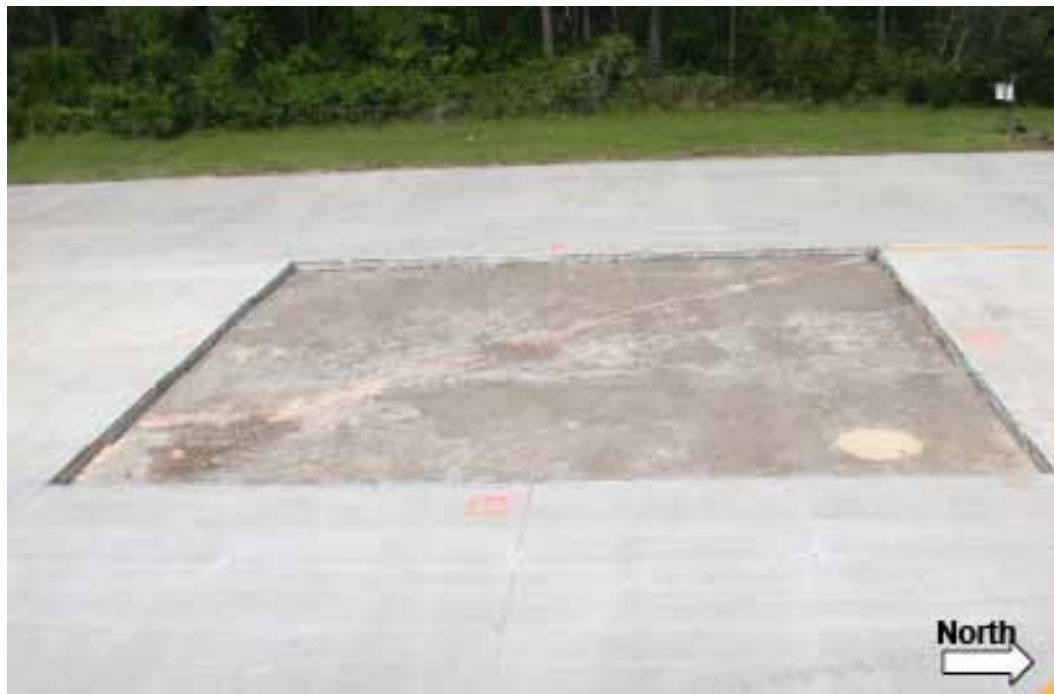
Figure 19. Crater 1 prior to cap placement.
