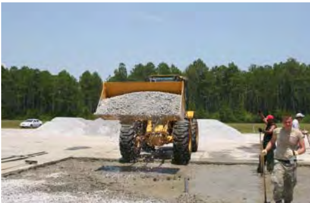
Figure 31. Adding stone to grout layer in Crater 1.
