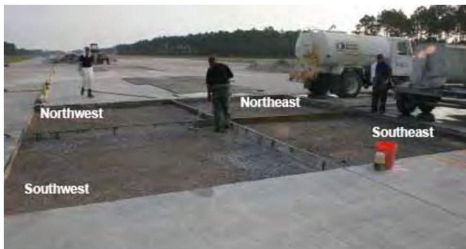
Figure 53. Formwork configuration in Crater 5.
