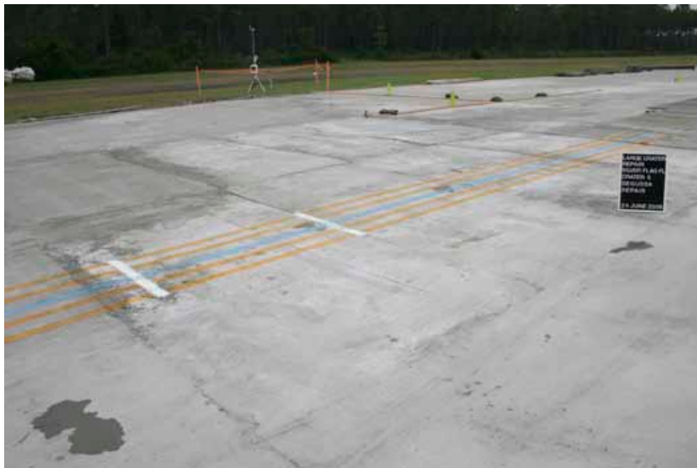
Figure 62. Final crater repair in Crater 5.
