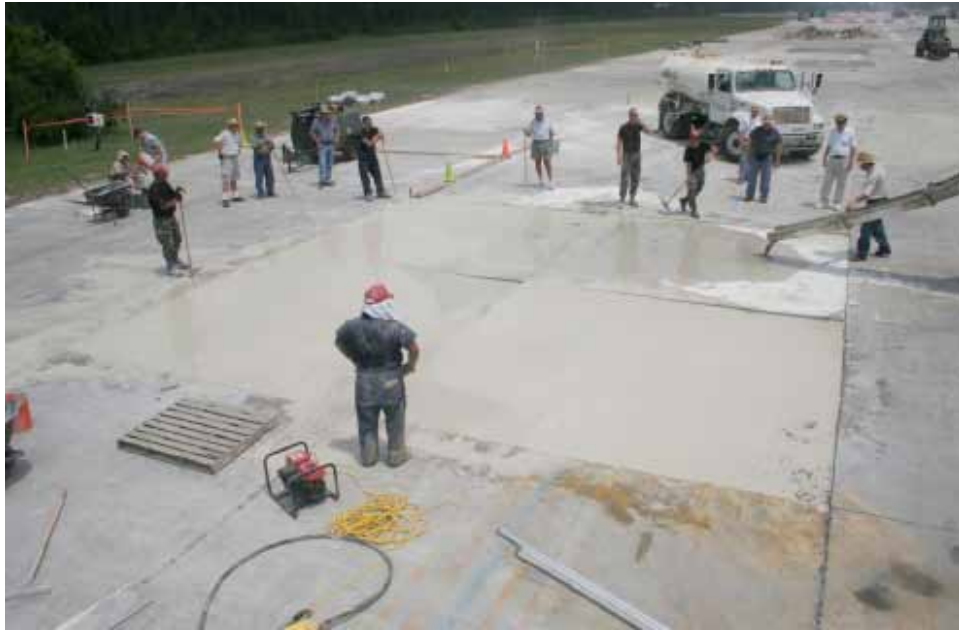
Figure 95. The repair material in Crater 3 is approximately 2 in below the existing pavement surface.
