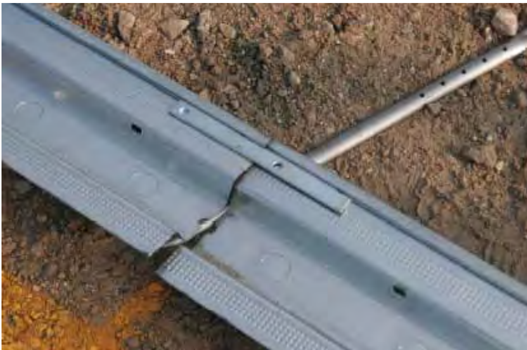
Figure 78. Stay-in-place aluminum forms with connecting tab used in Crater4 (Crater 3, too).
