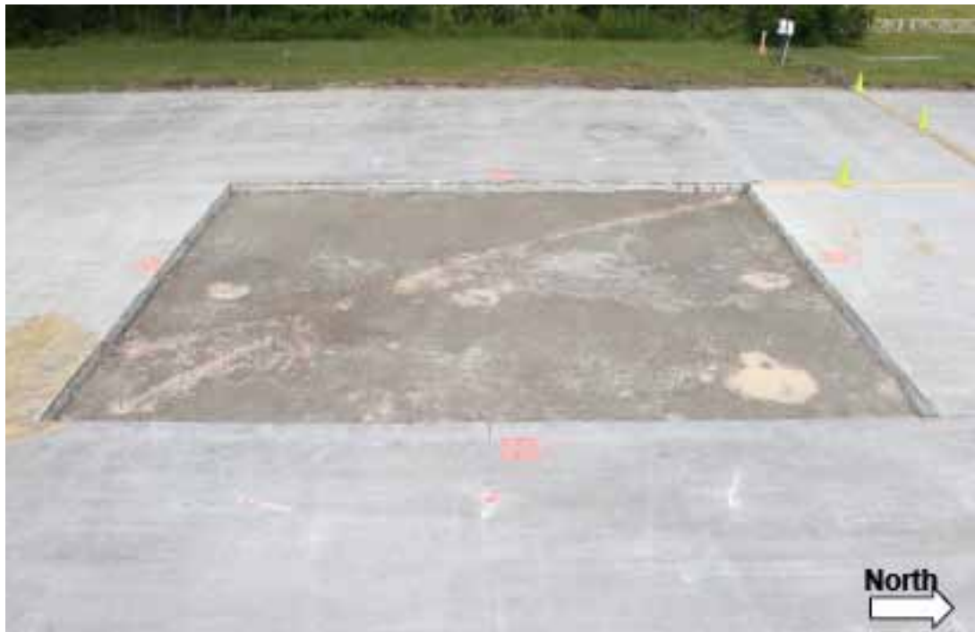
Figure 21. Crater 3 prior to cap placement.
