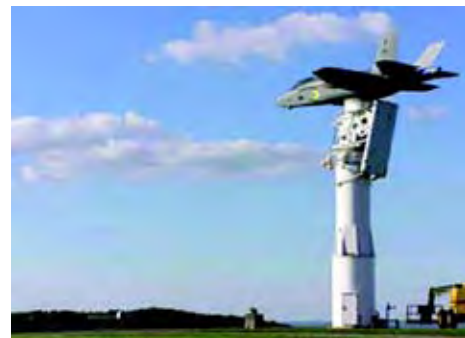
Newport Antenna Measurement and Research Facility
