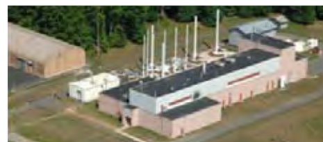
Bio Engineering Laboratory
