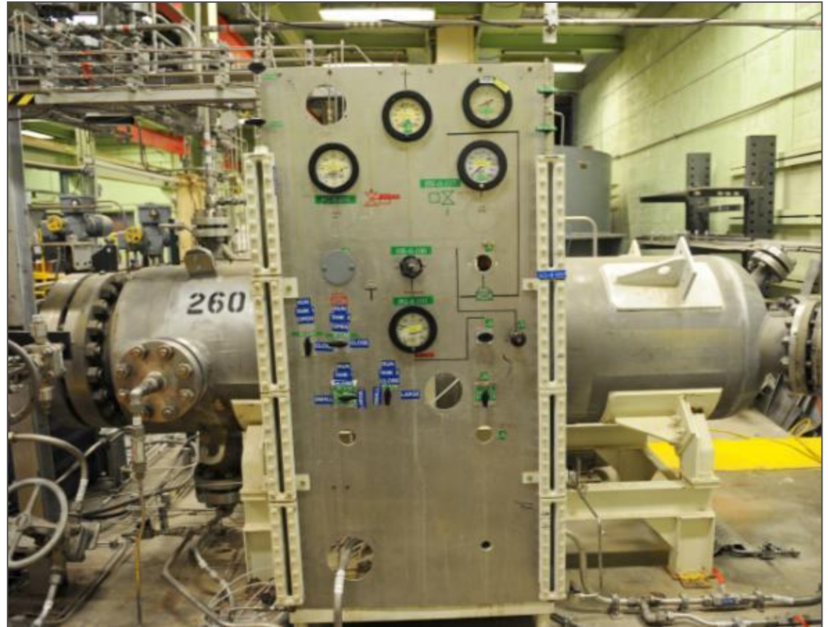
Fig14. Water Tank and Rear Pressure Regulator Panel (AFRL/RZOP, 2011)
