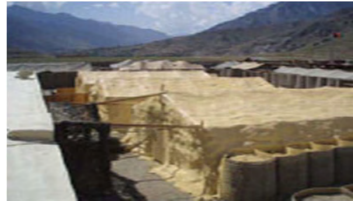
Foam insulation reducing heating and cooling from Net Zero Plus JCTD, used in Afghanistan and Iraq
