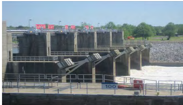
Figure 2. Supervisory Control and Data Acquisition and Hydromet Equipment for the Waterway at the Stennis Lock and Dam
