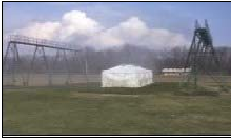
Figure 16. Rain Towers at Mile Loop.
