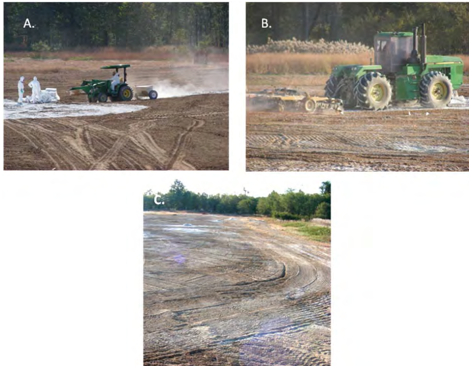
Figure 12. Topical application of the hydrated lime.
