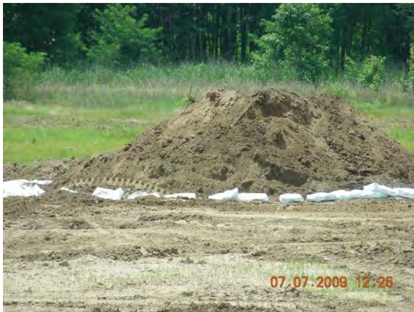
Figure 13. Illustration of lime application used in conjunction with detonations. Intact lime surrounding the mound is visible as white bags.
