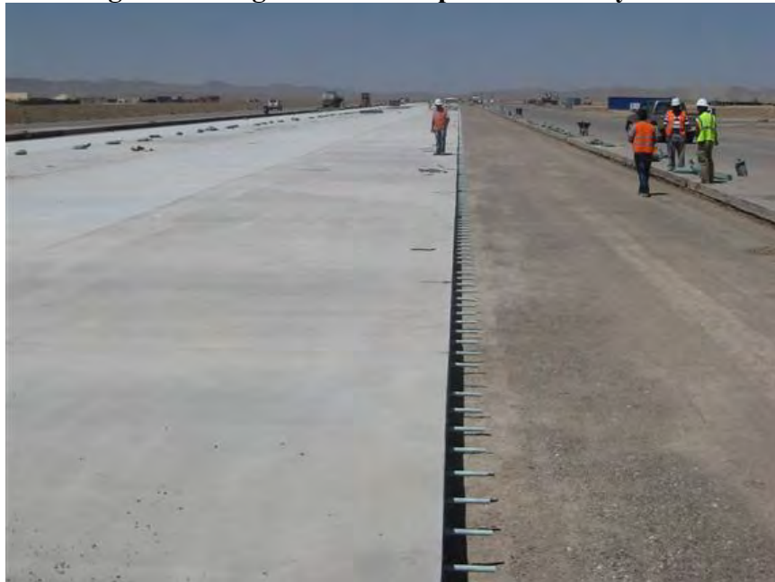
Figure 2. Progress on the Repair of Runway 18/36
