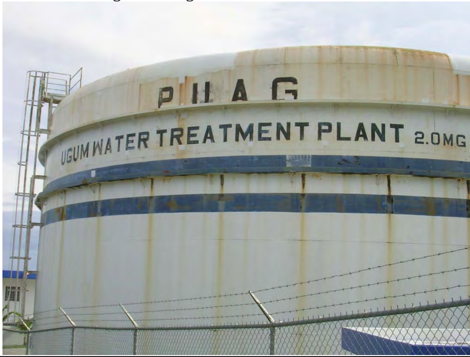
Figure 11. Ugum Water Treatment Plant
