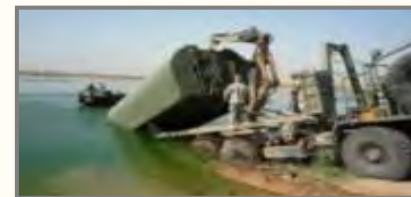
Improved Ribbon Bridge
