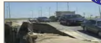
Dry Support Bridge
