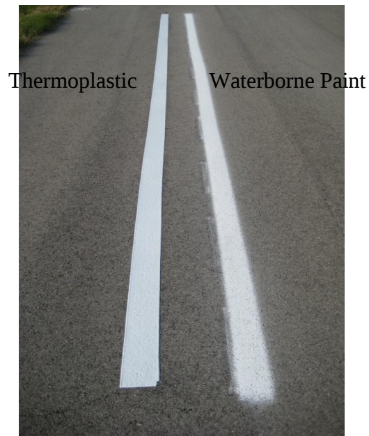
Figure 7: Sweeper Treatment Test Deck
