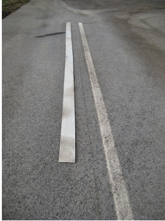
Figure 12: Thermoplastic Repositioned After Failure
