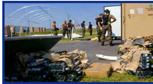
Civil Engineers Erecting shelters
