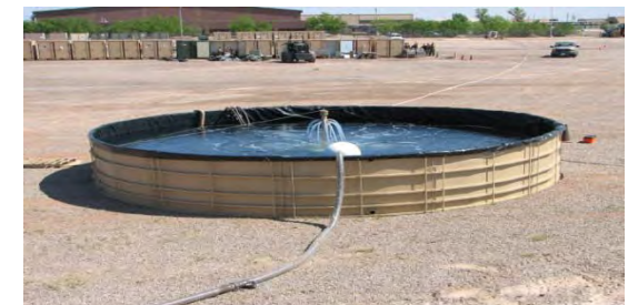
25K Gal Waste Tank with Aeration Unit
