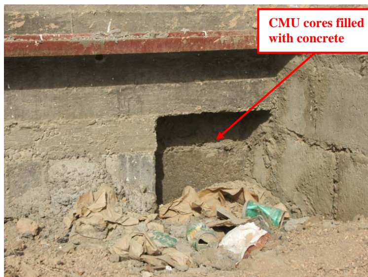
Site Photo 23. CMU cores filled with concrete
