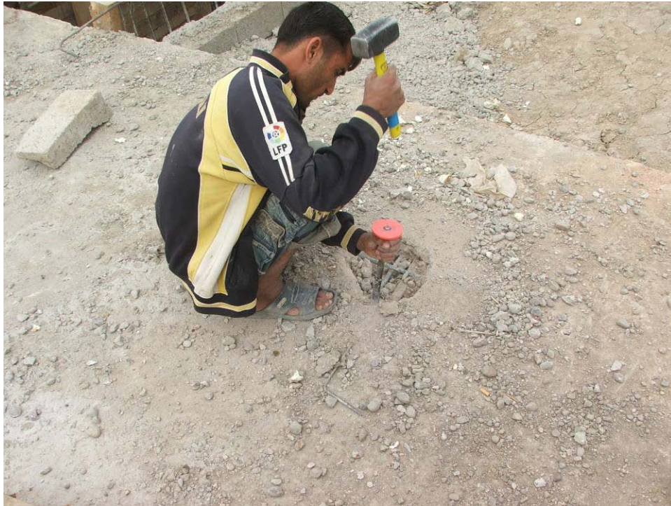
Site Photo 13. Chiseling tank lid for pipe penetration
