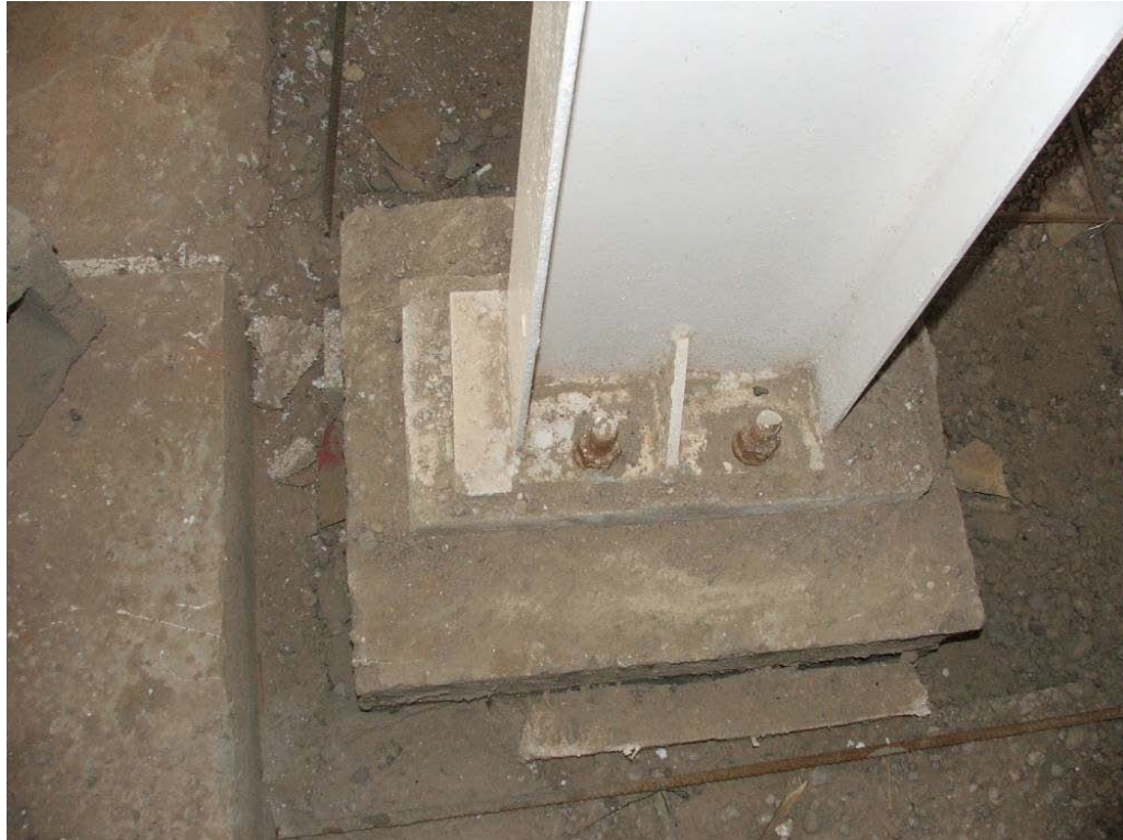
Site Photo 1. Typical foundation pedestal and anchor bolts
