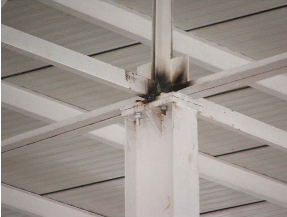
Site Photo 9. Lateral brace connection at column cap plate
