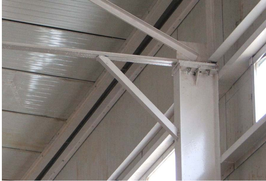
Site Photo 11. Diagonal brace from column to truss lower chord
