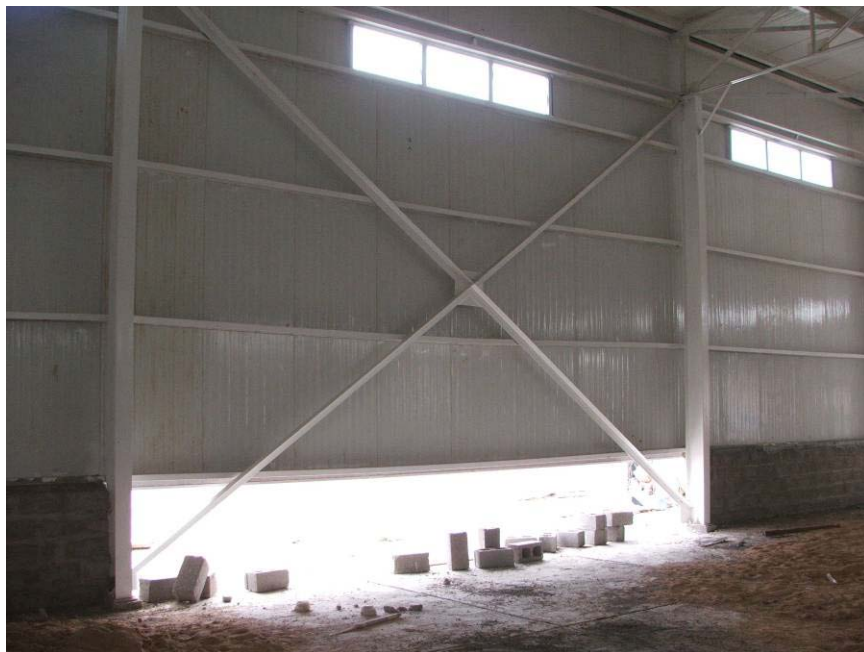
Site Photo 10. Lateral cross bracing between columns
