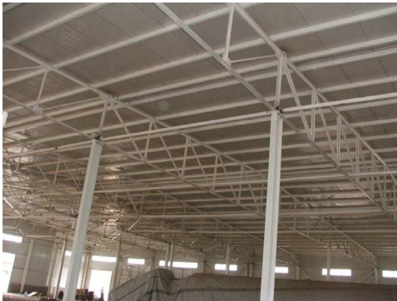
Site Photo 6. Lateral brace connection at column cap plate
