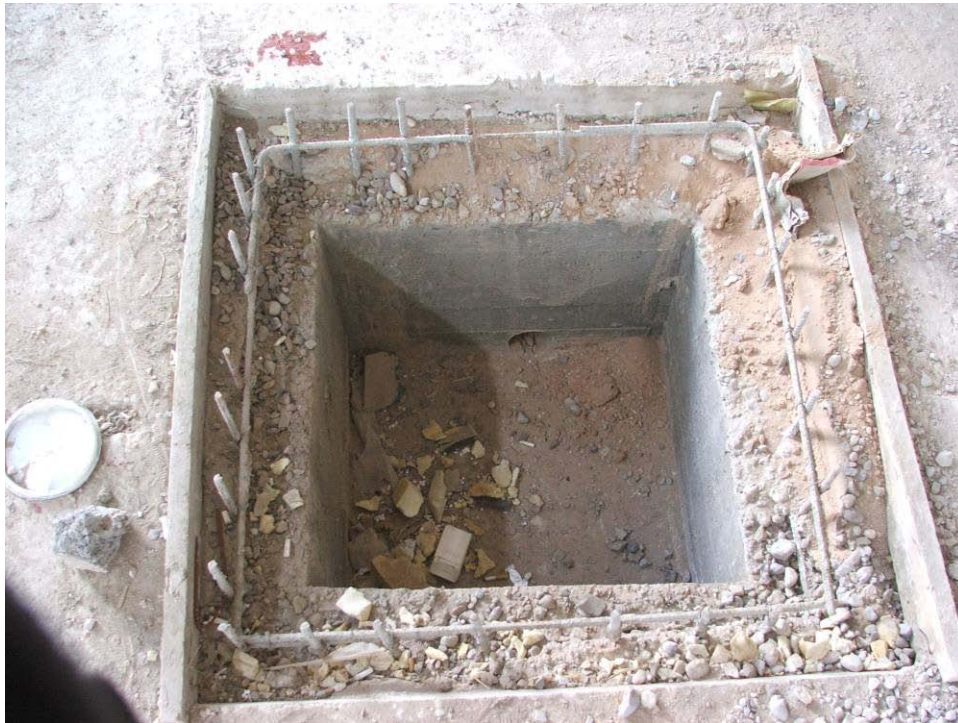
Site Photo 12. Cast-in-place sanitary sewer manhole
