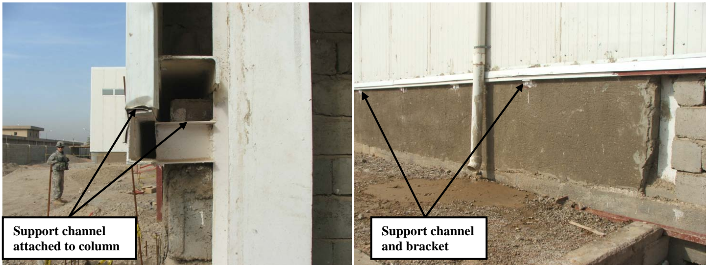
Site Photos 21 and 22. Support channel for sandwich panel
