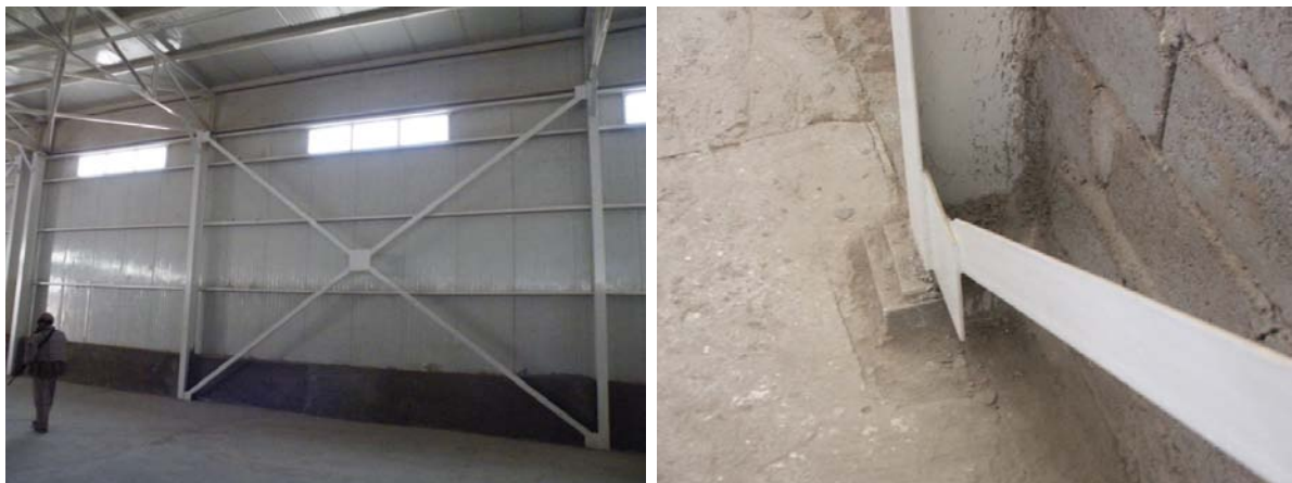
Site Photos 19 and 20. Cross bracing located to perimeter CMU wall interior
