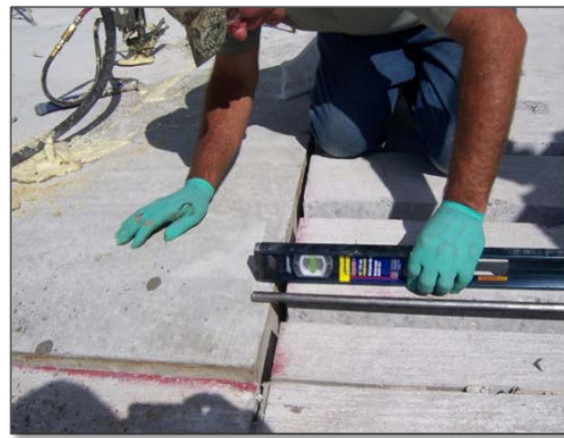
Leveling measurement
