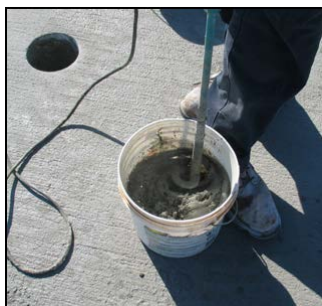
Mixing Pavemend 15.0™
