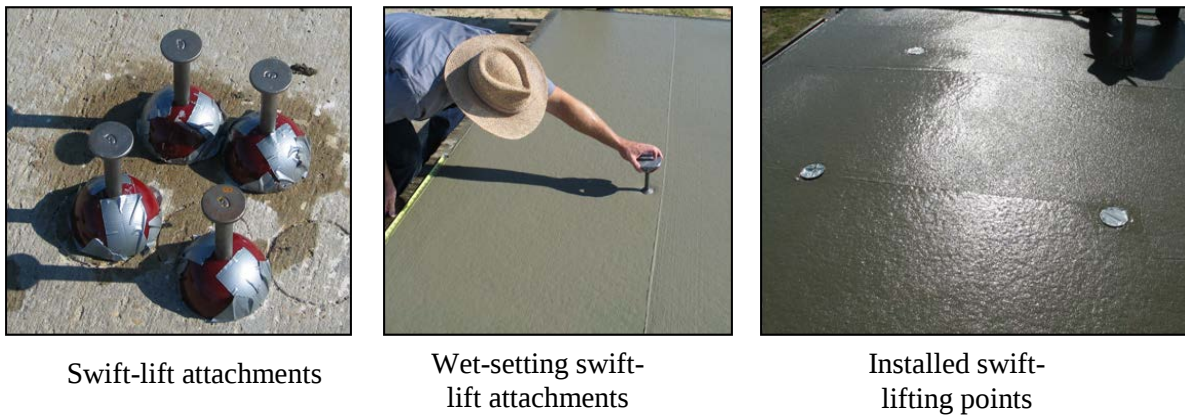
Figure 16. Swift-Lift Installation into Precast Concrete Panel
