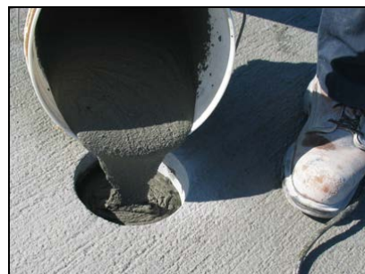
Placing Pavemend 15.0™
