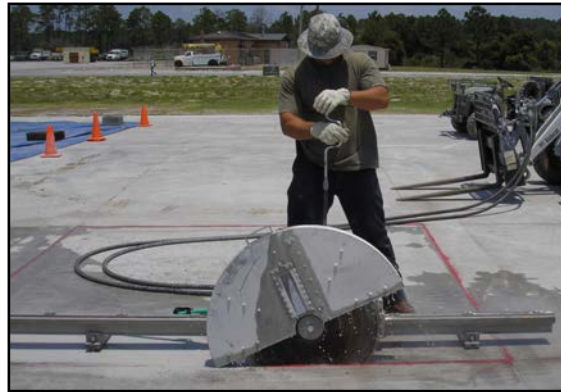
Figure 17. Wall-Saw Cutting Operation
