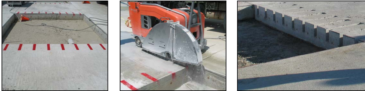
Figure 20. Dowel Slot Construction in the Existing PCC Slab
