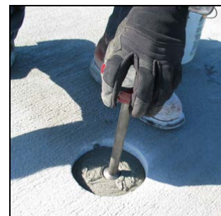
Installing lifting attachment
