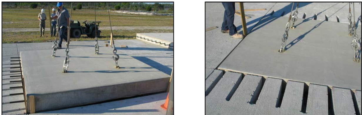
Figure 22. Precast Concrete Panel Placement Process
