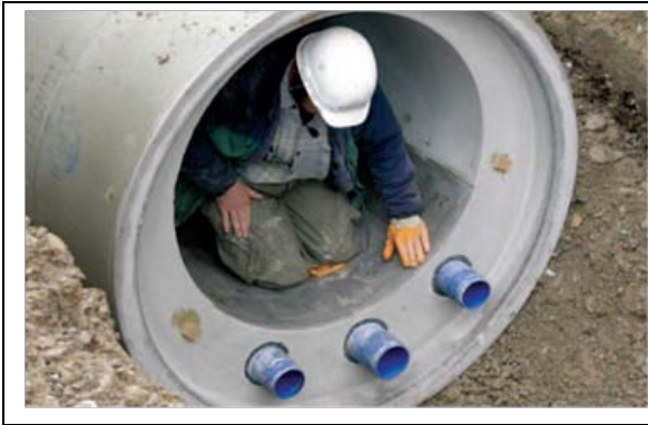
Figure B2. Integrated heat exchanger segment; (reference 2).
