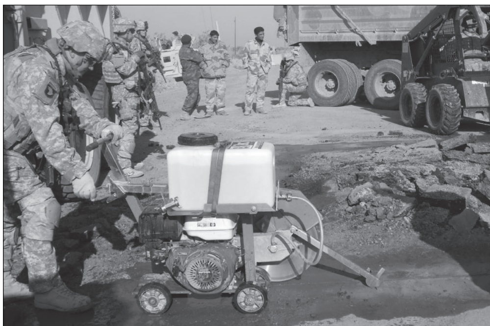
535th ESC Soldiers repair an IED crater.
