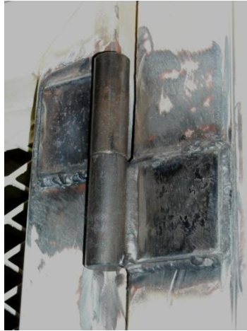
Figure 5. Subsequent Welding to the Cell Door
