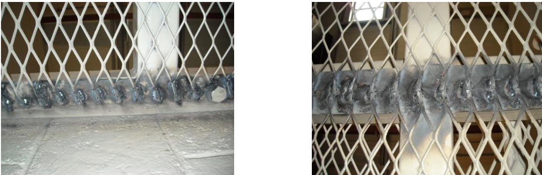
Figure 3. Re-Welded Cell Doors
