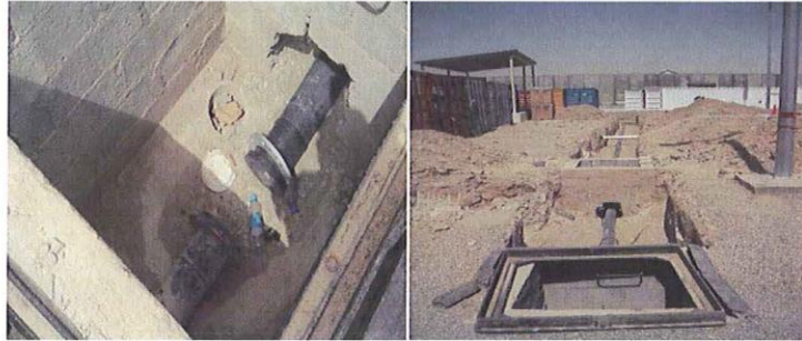
Figure 2. Main fire suppression lines being repaired.
