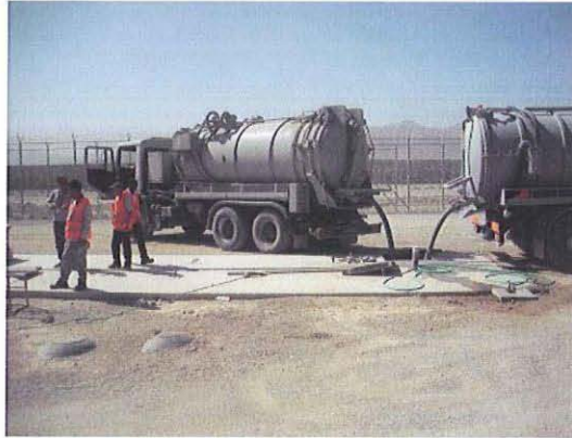
Figure 4. Contractor trucks removing sewage from DFIP lift stations.
