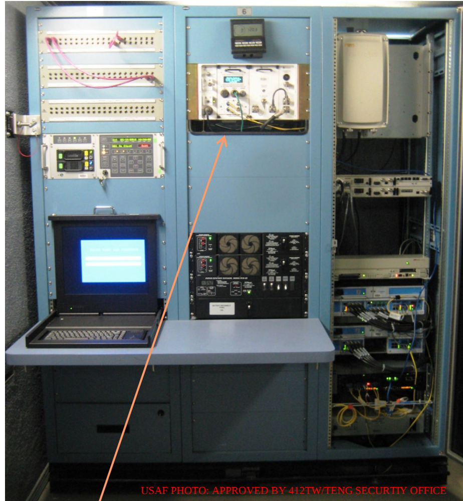
Ethernet/RS 422 Converter Added to Digital Microwave System For Remote Control of Radio
