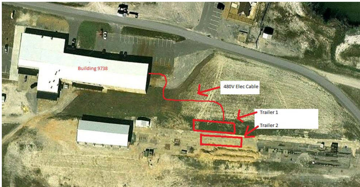
Figure 3: TWES Testing Location in relation to Building 9738
