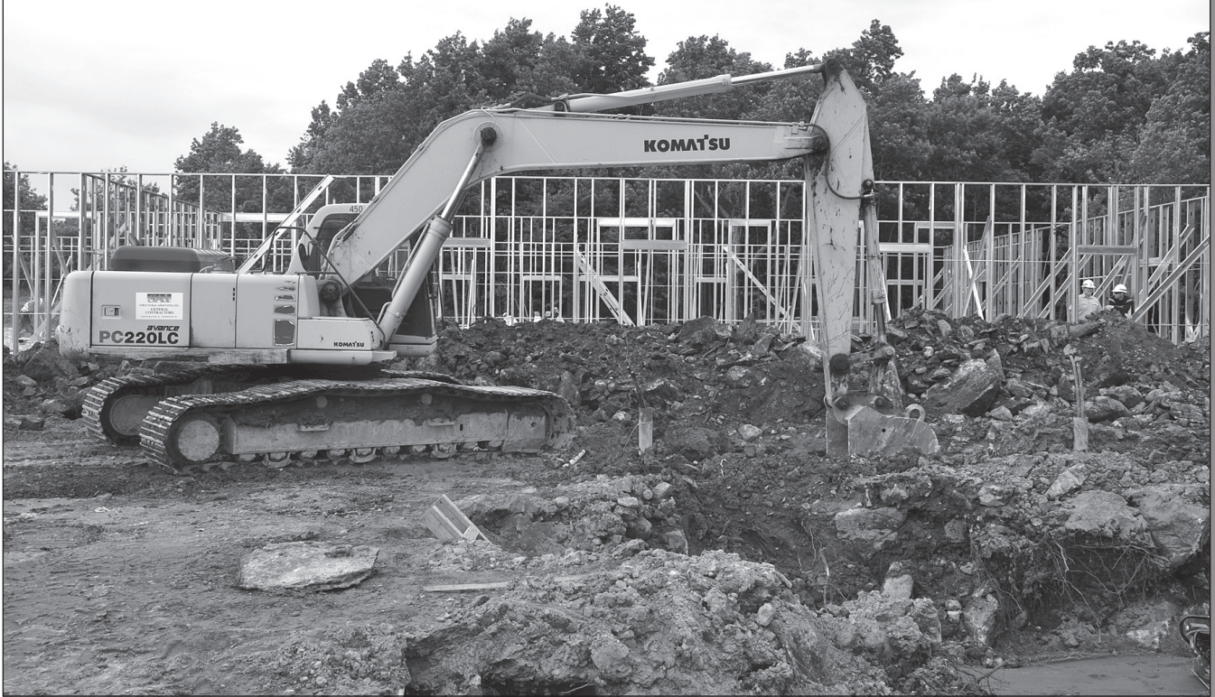
Crews work on trenches for geothermal wells, part of the heating and cooling system at the Fort Drum, New York, child development center.
