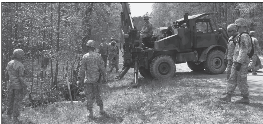
A small emplacement excavator pushes the pipeline through a culvert under a road.
