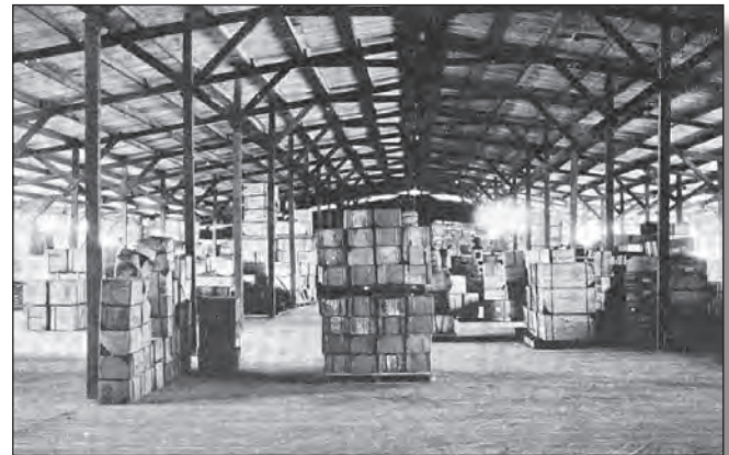
Figure 4. Prefabricated Storage Shed with Concrete Floor
