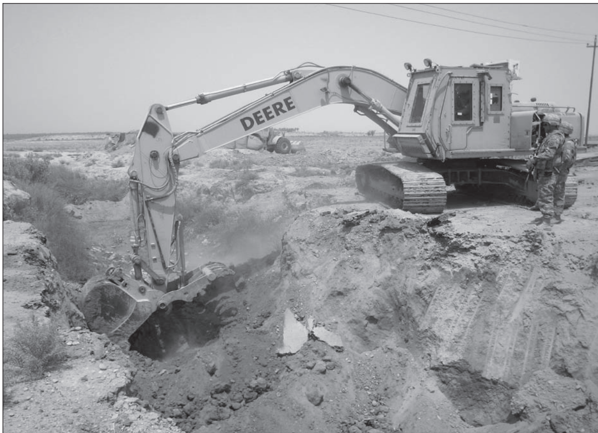
A Soldier excavates an area with a hydraulic excavator for the placement of a new culvert.
