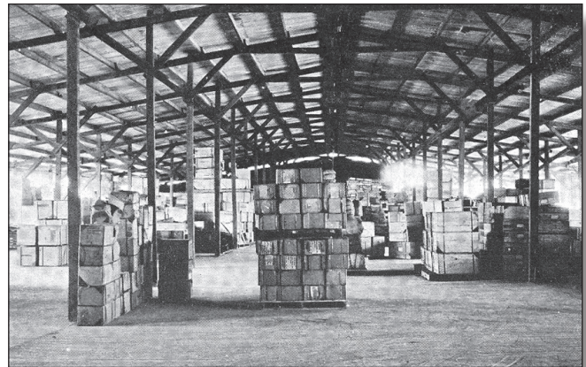
Figure 4. Prefabricated Storage Shed with Concrete Floor
