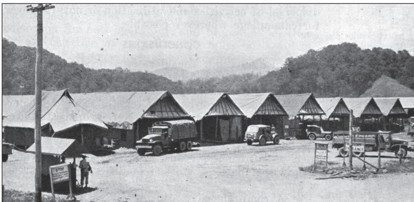
Figure 3. Storage Sheds, 20 Feet Wide, of Native Pole Construction
