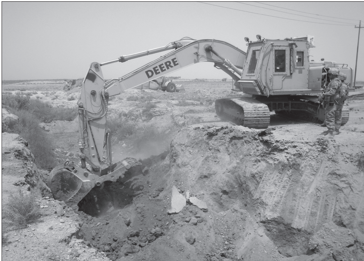
A Soldier excavates an area with a hydraulic excavator for the placement of a new culvert.
