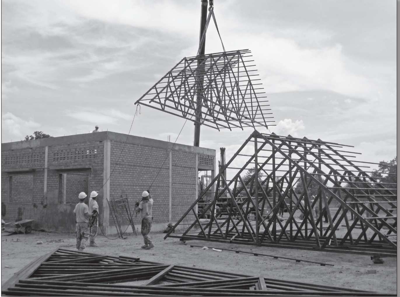
Soldiers guide a section of five trusses as a crane lifts it onto the schoolhouse roof.
