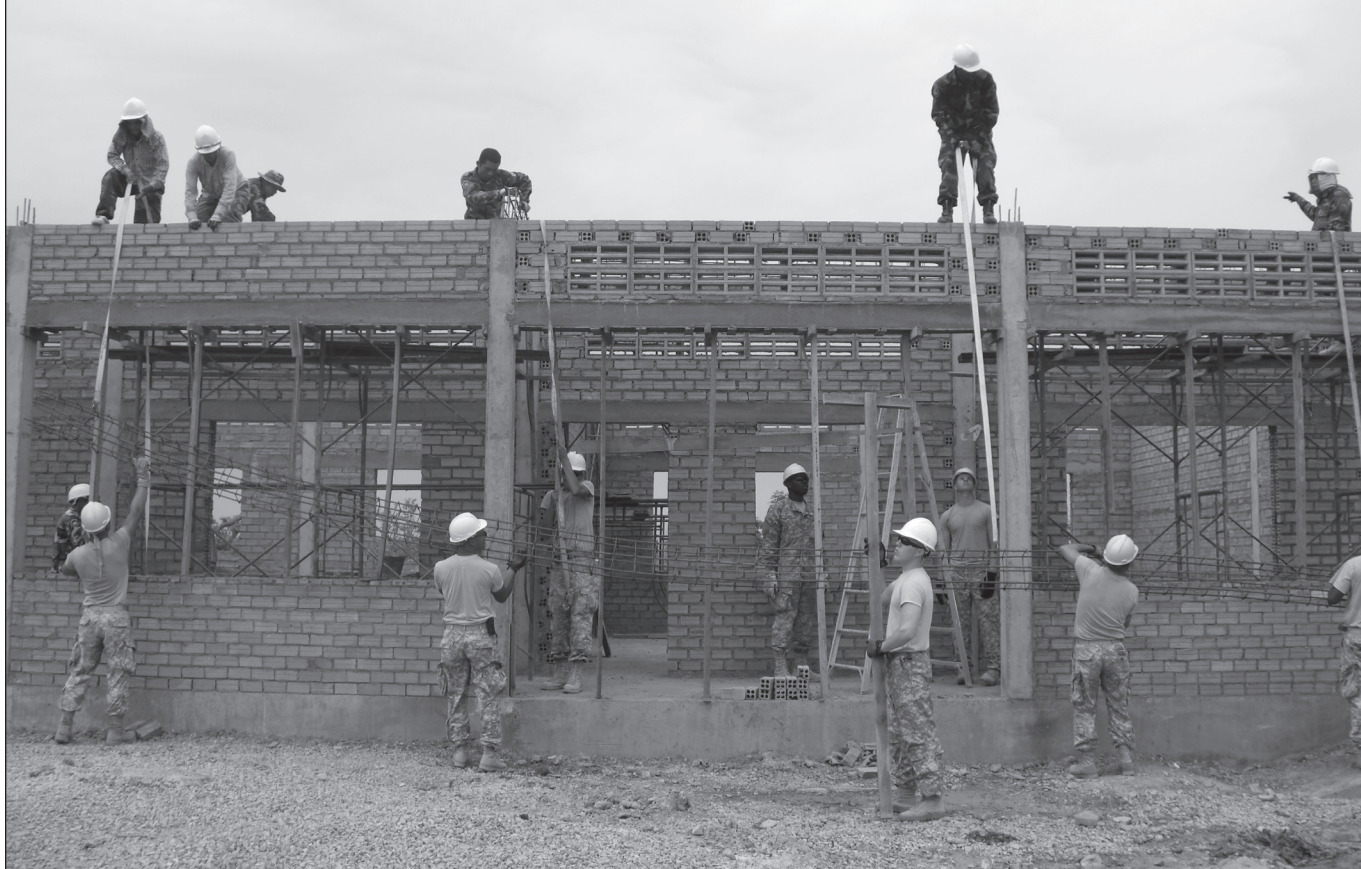
American and Cambodian engineers work together to lift rebar into place.
