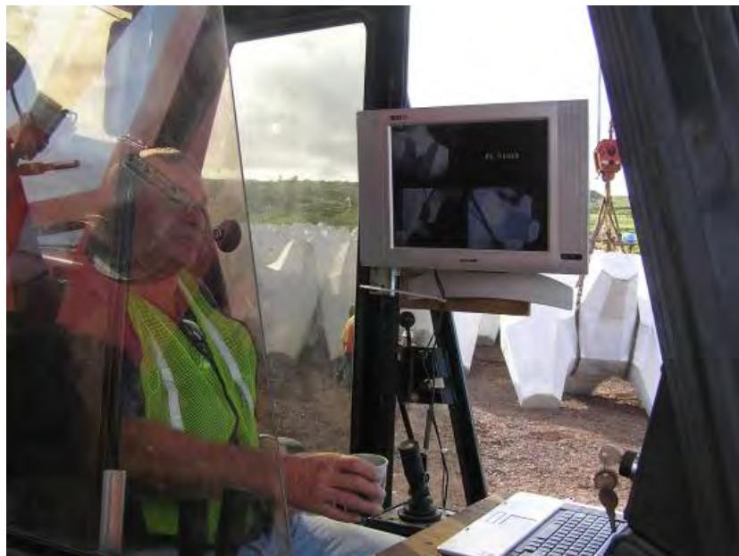
Figure 4.9. 4-way split screen for operator control of orientation and interlocking of armor units.
