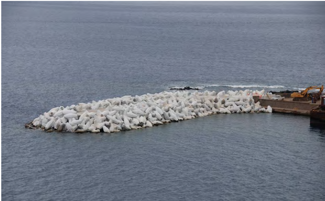
Figure 4.15. Harbor side of completed Kaumalapau Harbor breakwater rehabilitation with Core-Loc armor units (photo taken by Traylor Bros, Inc.).
