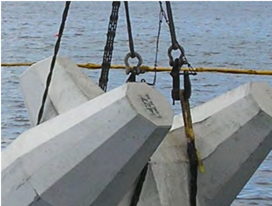
Figure 4.6. Double-sling with quick-release hooks for placing Core-Locs on the breakwater.
