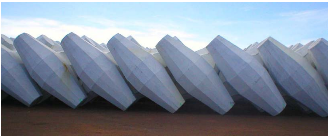
Figure 4.1. Core-Loc units at the storage yard on Island of Lanai, awaiting transport to Kaunapali Harbor breakwater construction site.
