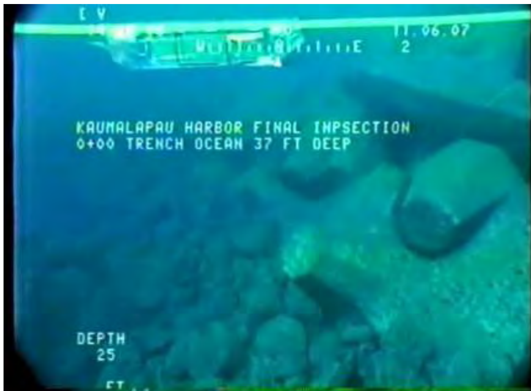
Figure 10.34. Ocean side trunk at approximately Station 0+00. Several toe units and interlocked units in the row above are visible at approximately 25-ft depth.
