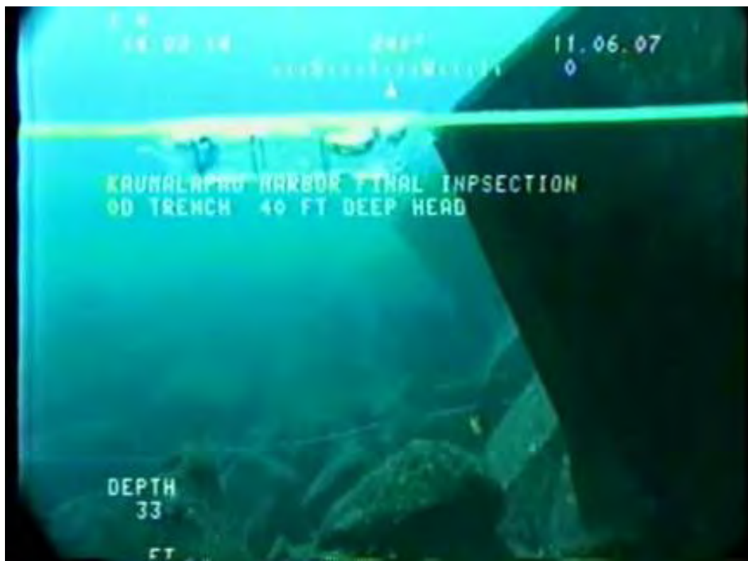
Figure 10.27. Breakwater head. Two well-entrenched toe units visible in “cannon” orientation.
