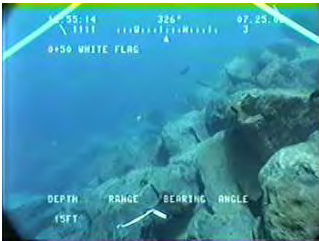
Figure 4.11. Use of ROV for underwater structure inspection of stone underlayer.
