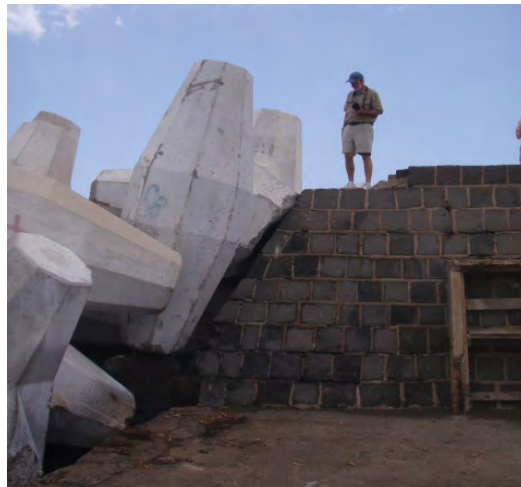
Figure 10.17. Photo from 2008 inspection showing side angle of harbor side tieback.
