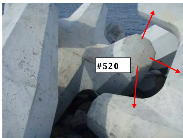
Figure 10.5. Poor contact between unit #520 and adjacent armor units at Station 1+36 on ocean side trunk (2007 photo). Unit #520 has moved 5.9 in. (15 cm) toward head from 2007-2010 (T-LiDAR).
