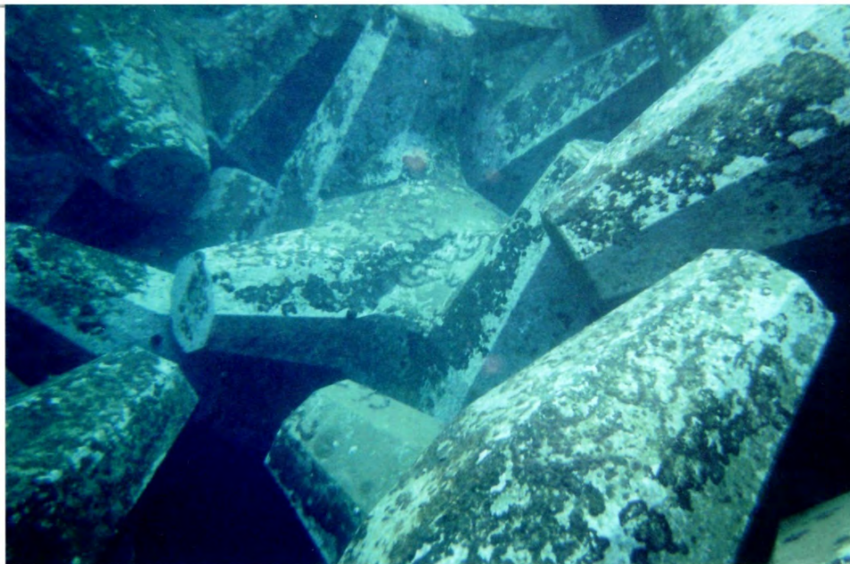
Figure 10.37. Photo of side slope armor units. No damage visible and well interlocked. (Photo by Orville T. Magoon, August 2009).
