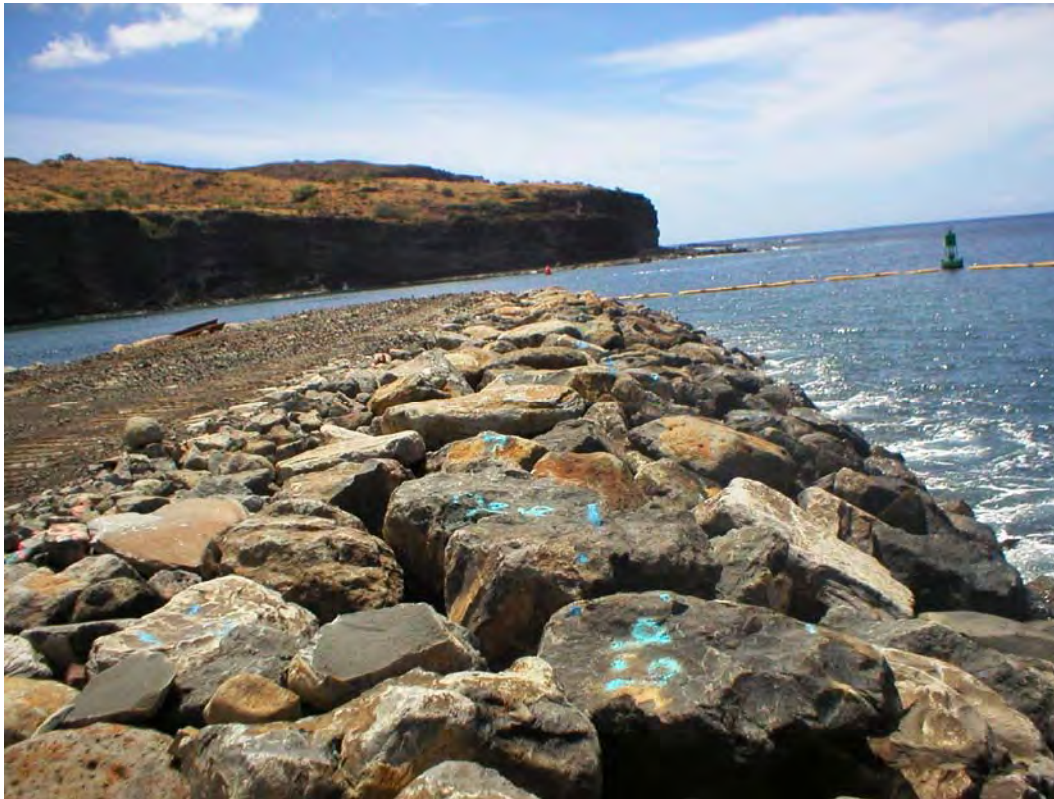
Figure 2.1. Breakwater underlayer prior to placement of Core-Loc armor layer.
