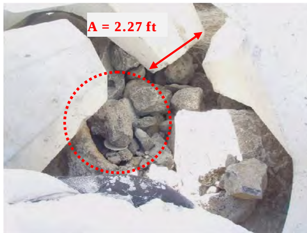
Figure 10.9. Undersize stone between ~0.5- to 2-ft diam, in void between armor layers and concrete cap on harbor side of breakwater head (2010 photo).
