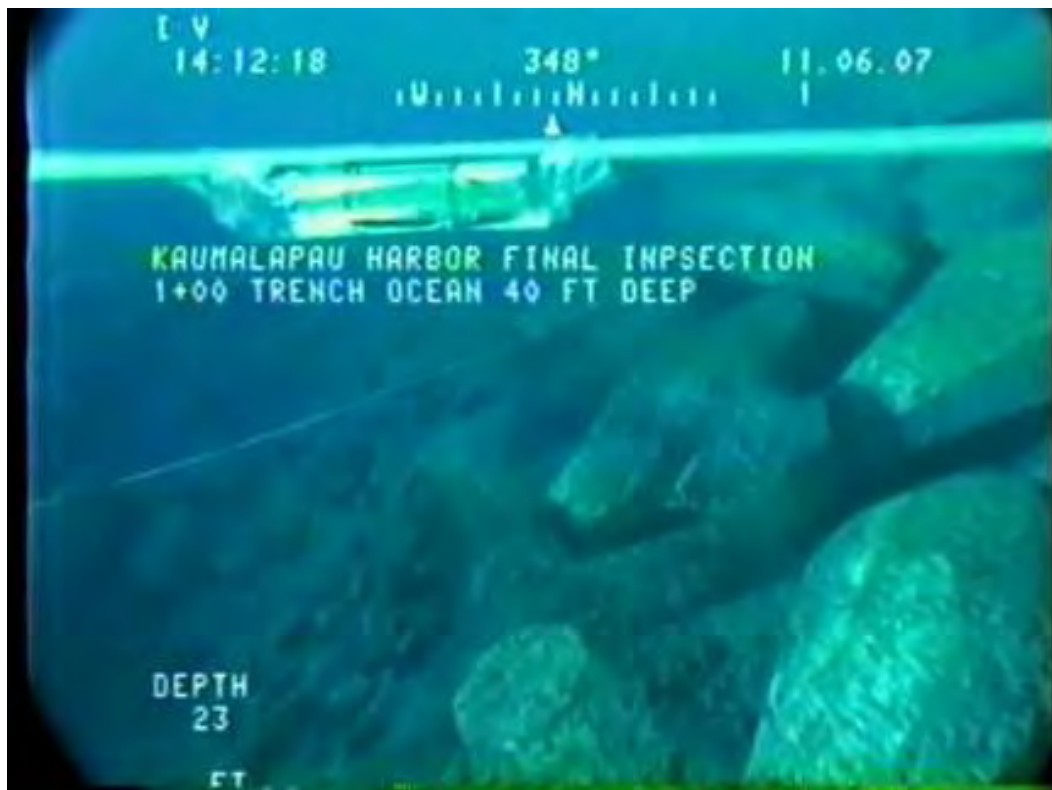
Figure 10.32. Ocean side trunk at approximately Station 1+00. Interlocking of armor units appears somewhat loose and toe trench appears to have widely varying stone sizes.
