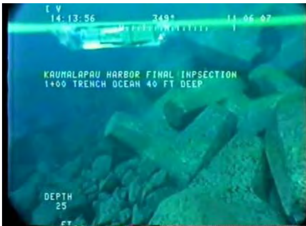
Figure 10.33. Ocean side trunk at approximately Station 0+50. Embedded toe unit in “cannon” orientation is visible with “straddled” unit directly above well interlocked.
