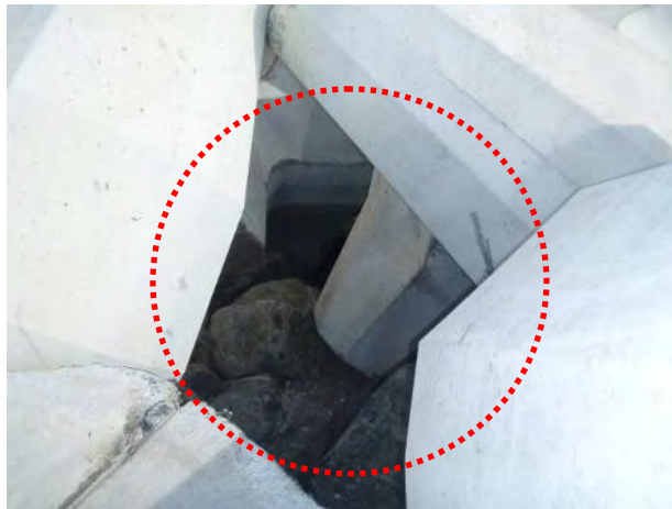
Figure 10.3. Void in armor layer on harbor side trunk at Station 1+59 with armor stone exposed. (2007 photo)
