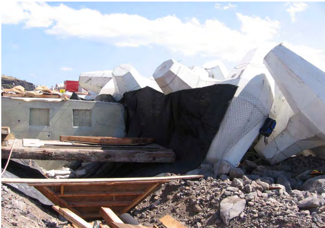
Figure 4.13. Breakwater crest cap segment being prepared, showing 3-ft-deep key trench into core material (Sea Engineering, Inc. and Group 70 International 2008).
