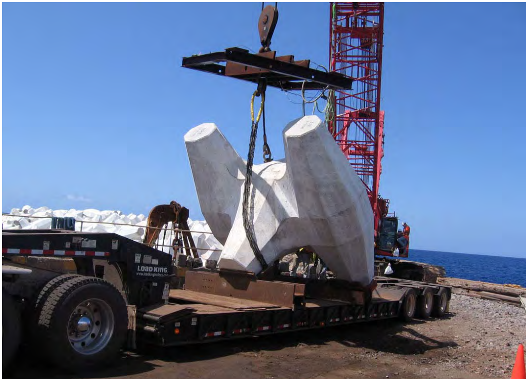
Figure 4.2. Core-Loc unit rigged for offloading at the breakwater construction site after being transported from the storage yard (Sea Engineering, Inc. and Group 70 International 2008).
