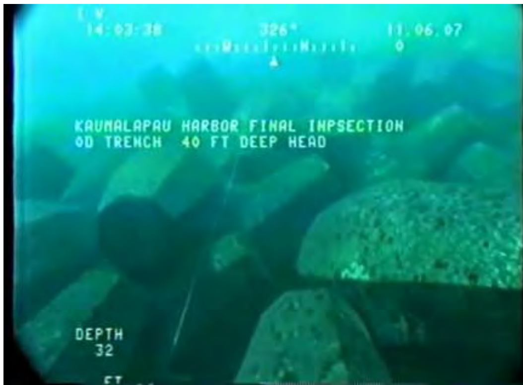
Figure 10.28. Ocean side of breakwater head. Side slope of breakwater shown with armor units well interlocked.
