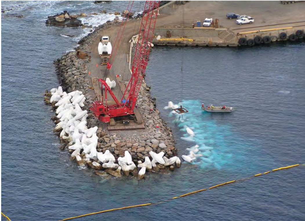
Figure 4.5. GPS placement of Core-Loc armor units on Kaumalapau Harbor breakwater during rehabilitation.
