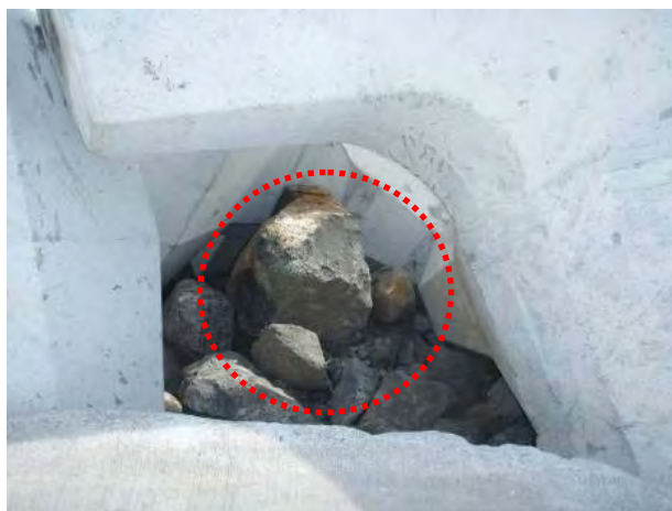
Figure 10.10. Undersize underlayer stone on harbor side trunk at Station 1+51, estimated to be ~0.8- to 2.5-ft diam. (2007 photo)
