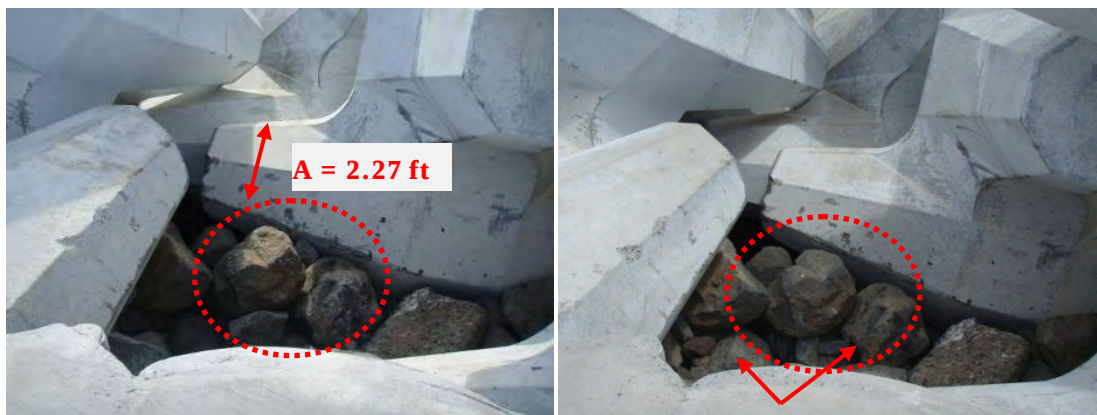
Figure 10.8. 2007 photo of undersized stone between ~0.8- and 2.5-ft diam, near crest on harbor side of breakwater head (left). 2009 photo of same location with noticeable changes including broken stones and additional small stones indicated by arrows (right).
