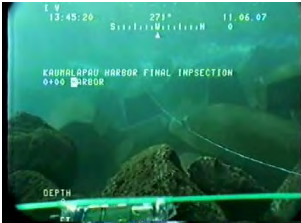
Figure 10.22. Harbor side root and tieback at approximate Station 0+00. Armor units in background and stone toe berm in foreground.
