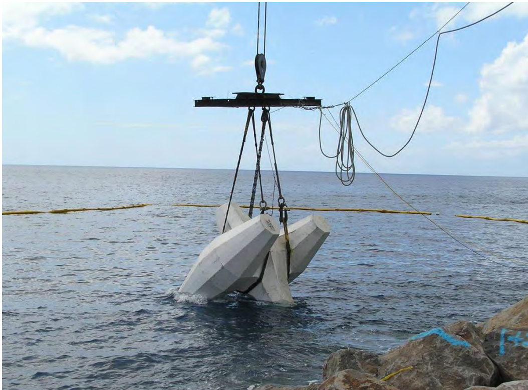
Figure 4.7. Lifting frame with tugger cables attached to double-sling for precise placement of Core-Loc units on the breakwater (Hays, Smith, and Sullivan 2006).
