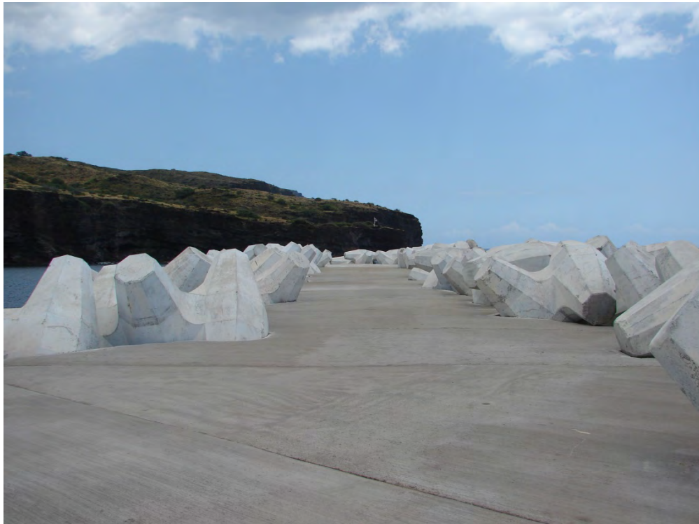
Figure 4.14. Completed breakwater crest cap.
