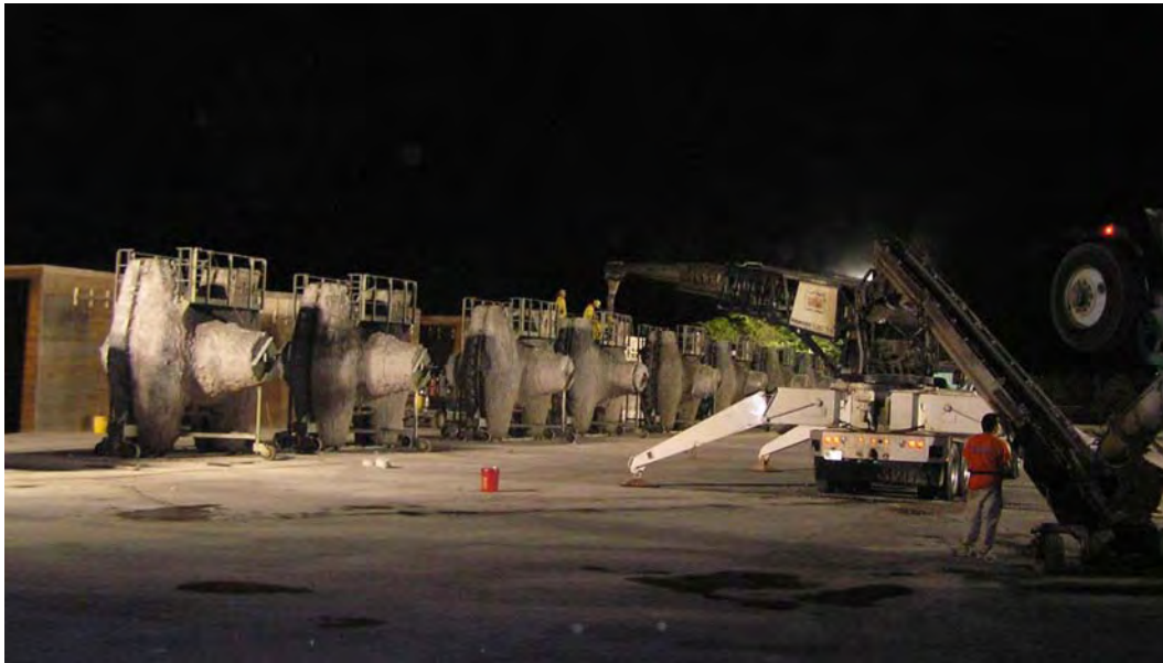
Figure 3.5. Casting concrete Core-Loc armor units at night for better temperature control.
