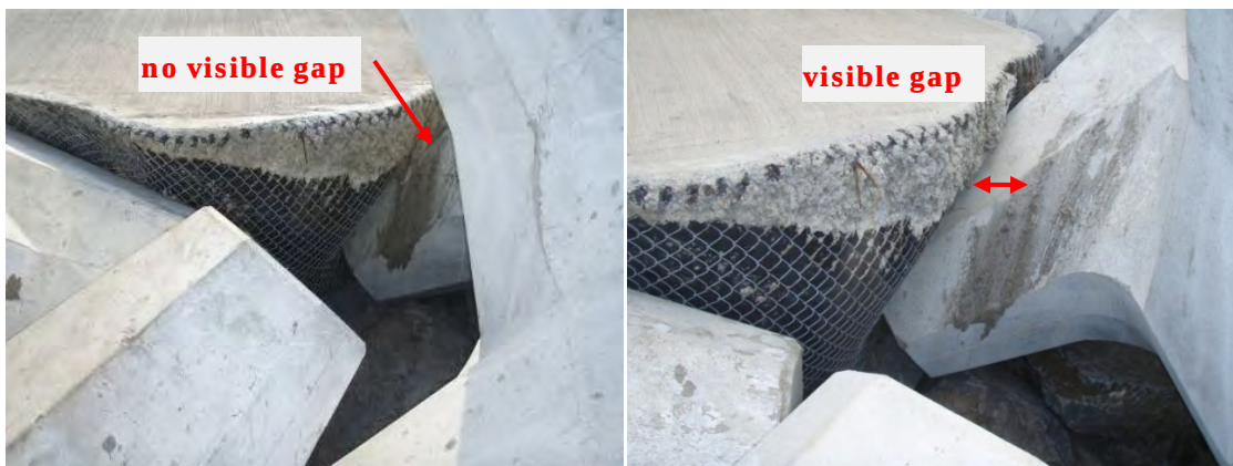
Figure 10.15. Exposed edge of concrete cap with apparent pulling away of armor unit between 2007 (left) and 2009 (right) on ocean side trunk at Station -0+14.
