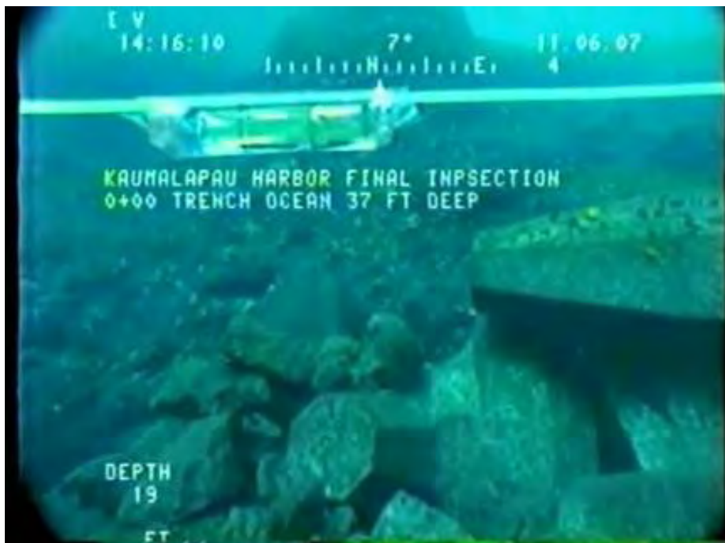
Figure 10.35. Ocean side root. Tieback of armor layer into reef platform appears flush. Scattered armor stones from toe trench or stone buttress visible near tieback.
