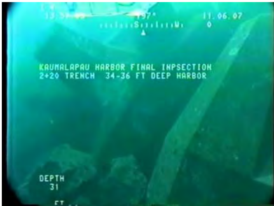
Figure 10.26. Harbor side head at approximately Station 2+20. Toe units in “cannon” orientation are visible at approximately 31-ft depth.
