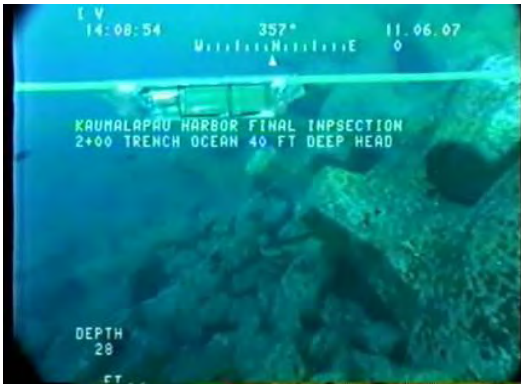
Figure 10.30. Ocean side trunk at approximately Station 2+00. Toe armor units and second row of armor units visible. Slope of toe trench/stone buttress appears somewhat steep.
