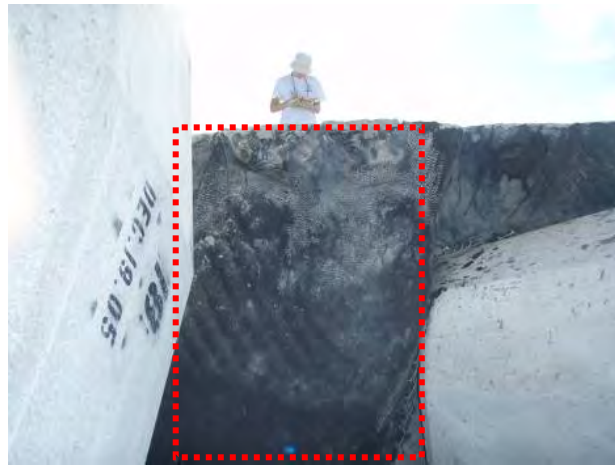
Figure 10.11. Exposed underside of concrete cap at Station -0+28 along ocean side trunk.
