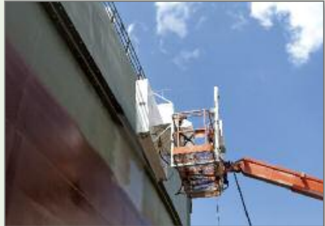
A painter operates the enclosure on its first paint run.
