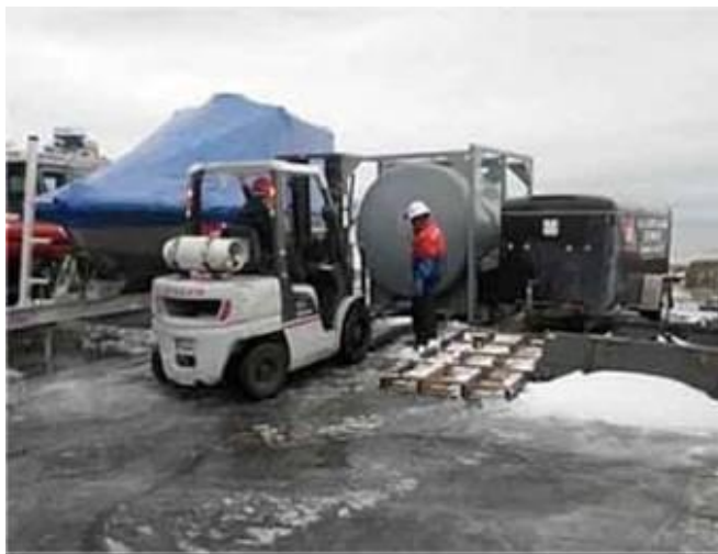
Figure 2. Aborted attempt by small forklift to move empty oil collection storage tank.
