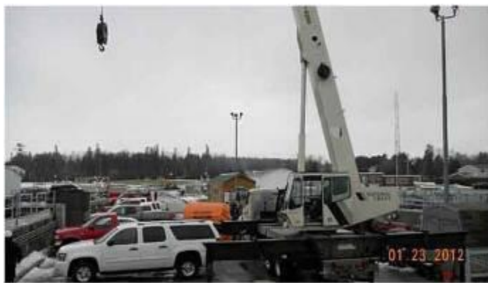
Figure 1. Crowded loading area makes load-out difficult.
