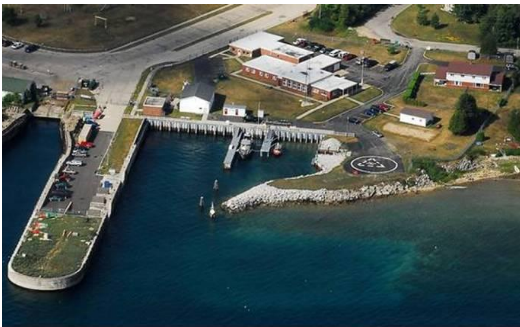
Figure F-3. CG Station St. Ignace pier (staging location).
