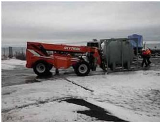
Figure 3. Appropriate-sized forklift moving empty oil collection storage tank.
