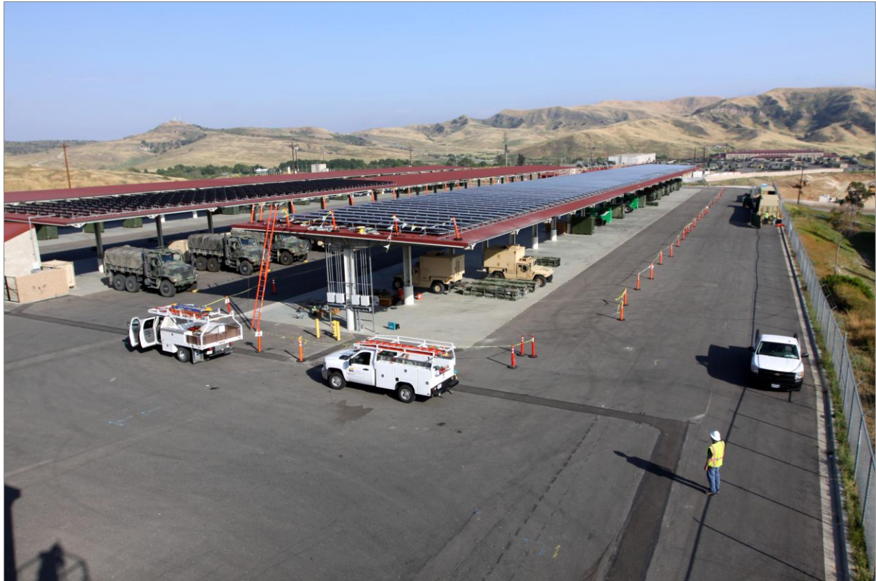
Solar panel installation at a Las Pulgas artillery shelter nears completion as contracted workers finish setting up 672 modules at MCB Camp Pendleton. Photo taken by Lance Cpl. Daniel Boothe on 5/15/2010 Source: Defense Imagery
