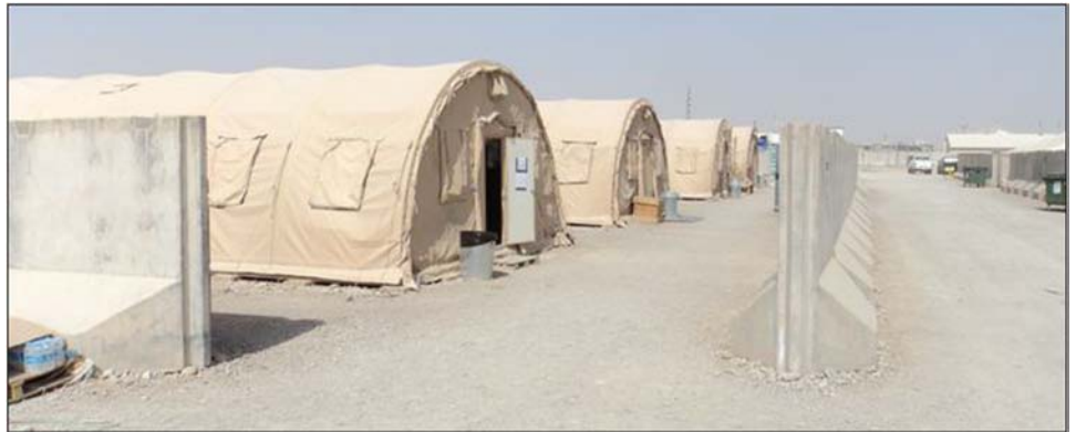
Figure 4: Expeditionary Living Facilities at Camp Leatherneck without DOD-recommended Solar Shading
