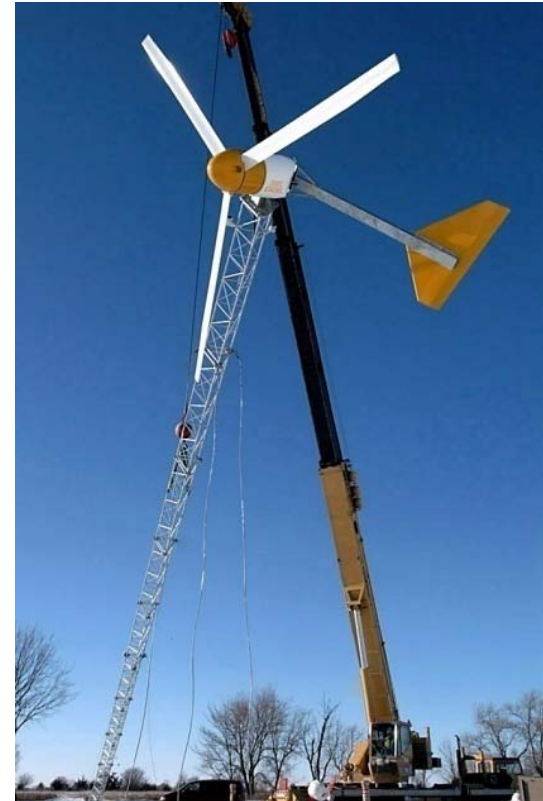
10-kW turbine for ground water circulation, reducing grid electricity consumption by 26% at former Nebraska ordnance plant
