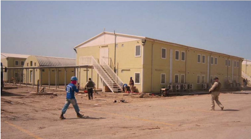
The ISFF-funded Federal Police Sustainment Brigade complex in Baghdad is now scheduled for completion in August 2012. (USACE photo)
