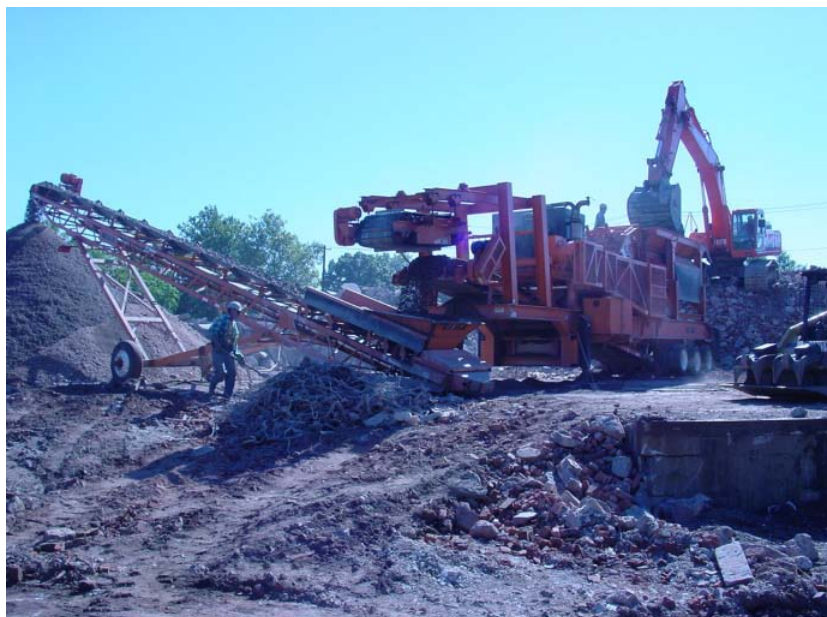
Figure B8. Crushing material at former GAF site.
