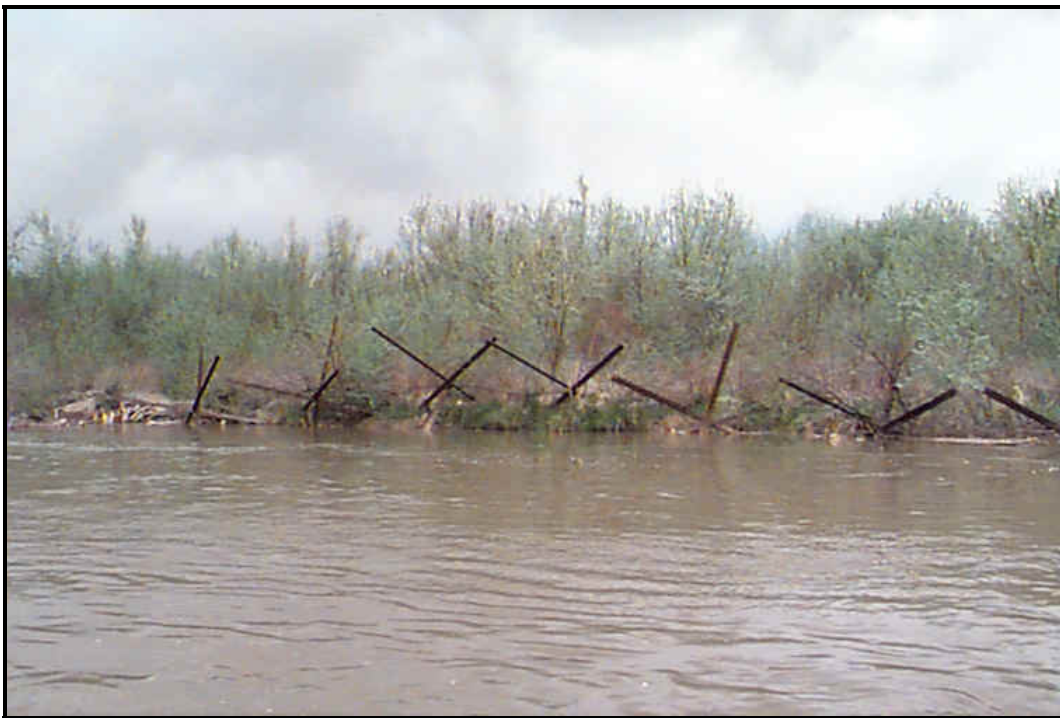
Figure 27. Jetty jacks lined along the bank of the Rio Grande trap sediment and plant material during flooding events, and have stabilized over-bank areas over the course of several years.
